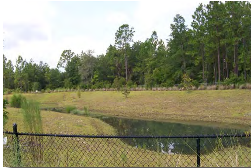
On-site stormwater management
