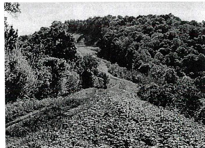
These images are of the TL-585 pipeline in Kanawha County, WV, undergoing restoration. The ridgelines are fully restored back to original contours and native vegetation has been used to stabilize the soil.
