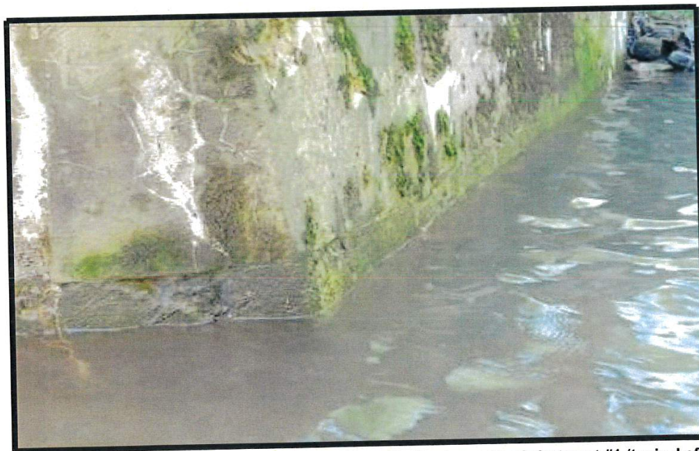
Light scaling along the base of the breastwall and both wingwalls of abutment #1 (typical of abutment #2).
