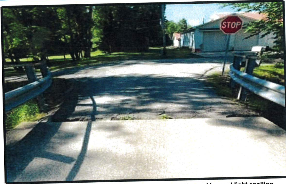
Condition of the approach at abutment #1, with moderate cracking and light spalling.
