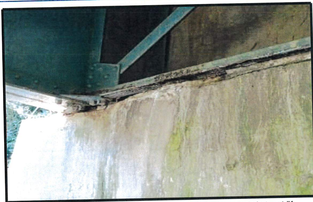
Light to moderate spalling along the front edge of the bridge seat at abutment #1.
