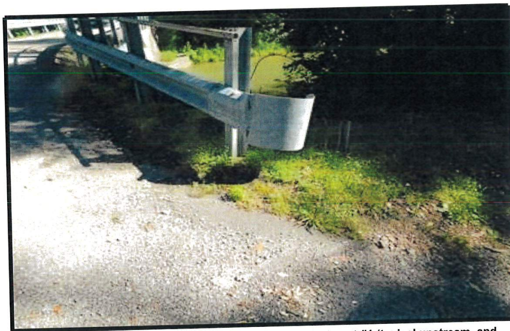
Minor damage on the downstream buffer end near abutment #1 (typical upstream, and downstream at abutment #2).
