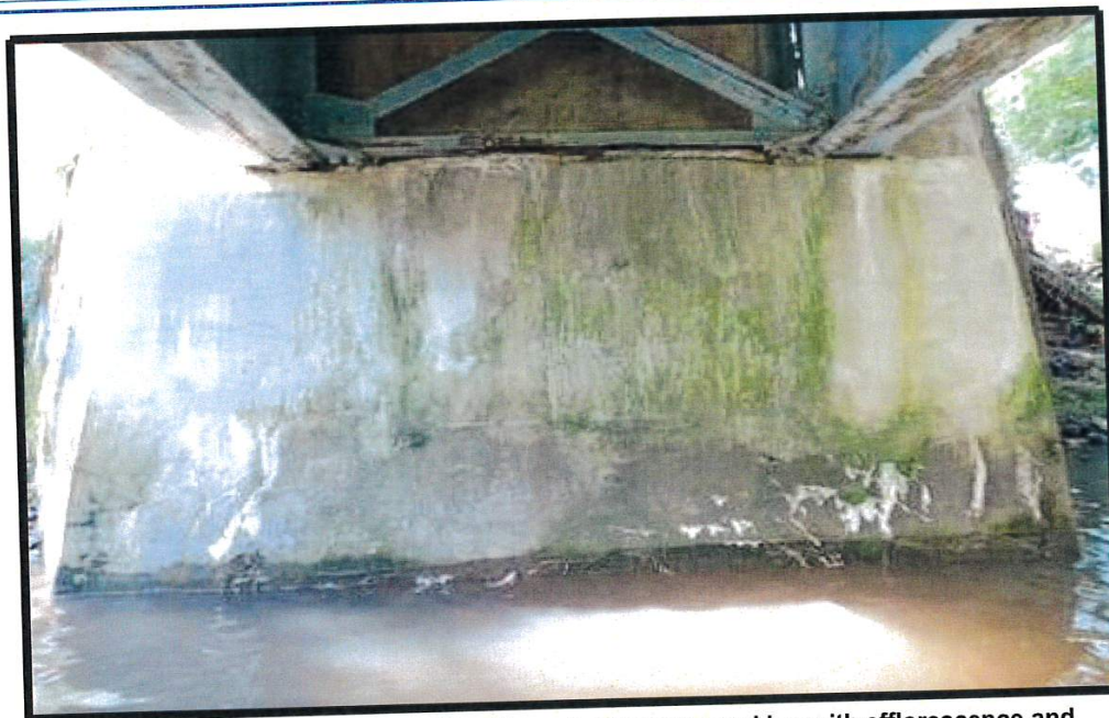
Overall condition of abutment #1, with moderate map cracking with efflorescence and patching (typical of abutment #2).
