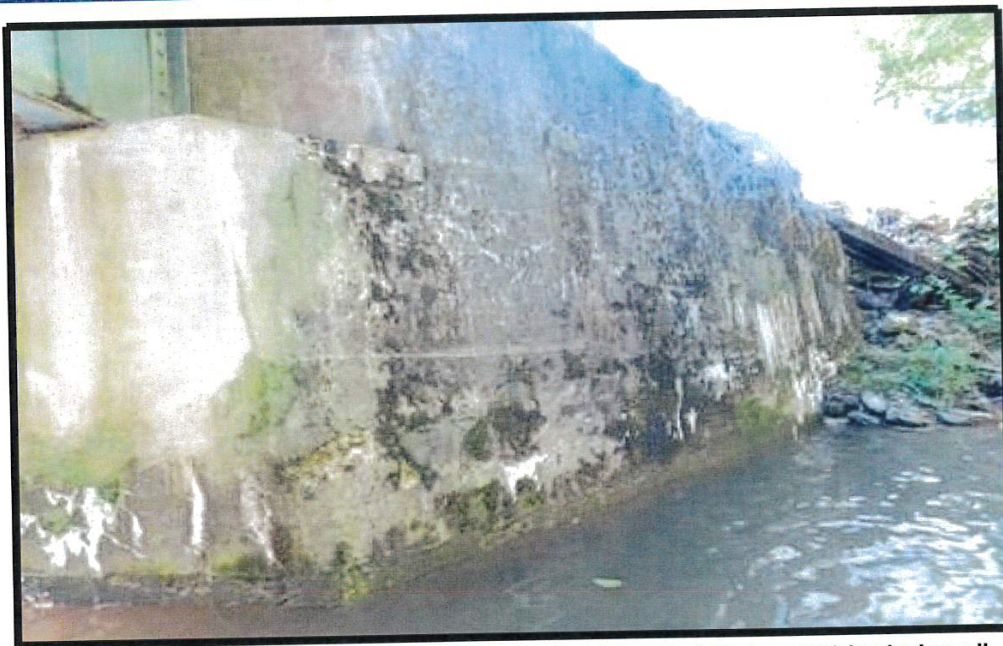
Minor spalling with efflorescence on the upstream wingwall of abutment #1 (typical on all four wingwalls).
