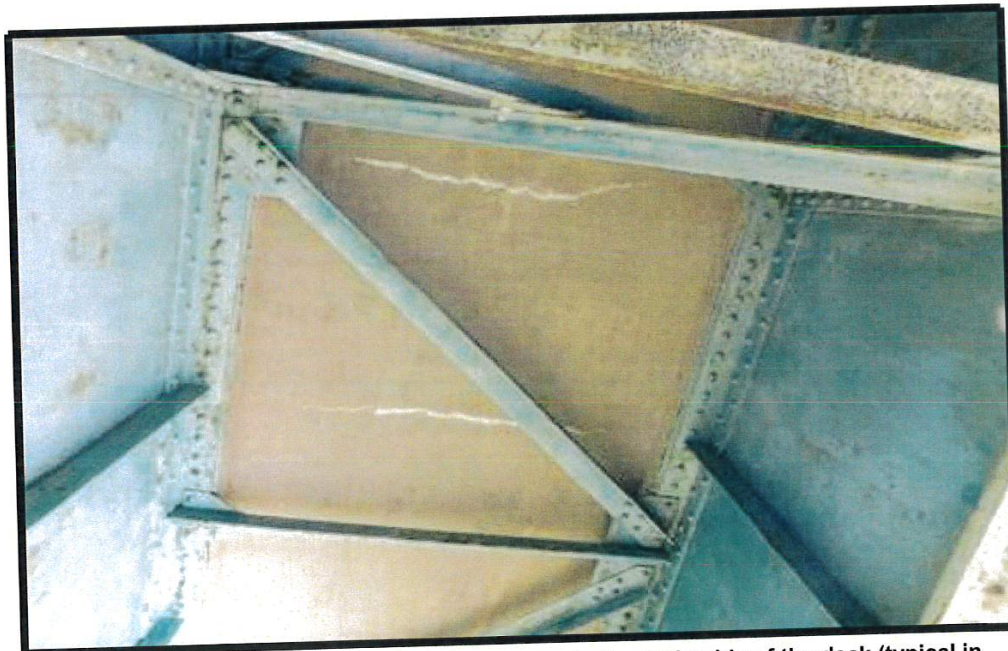
Transverse hairline cracking with efflorescence in the underside of the deck (typical in multiple locations).
