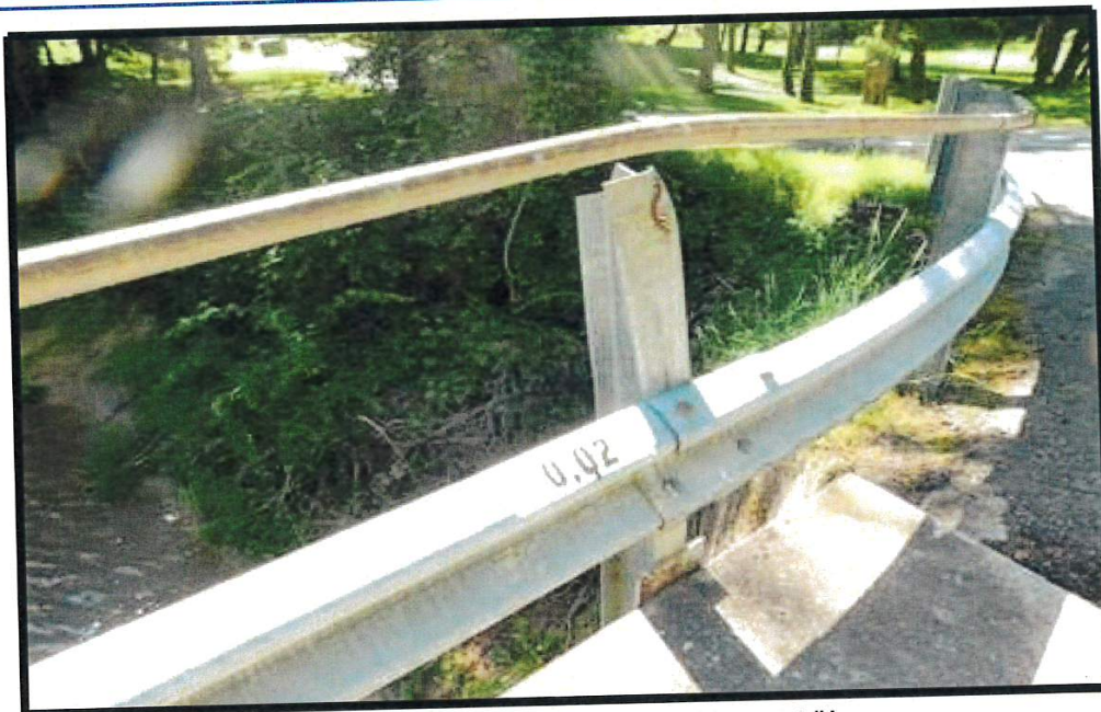
Damaged handrail downstream at abutment #1.
