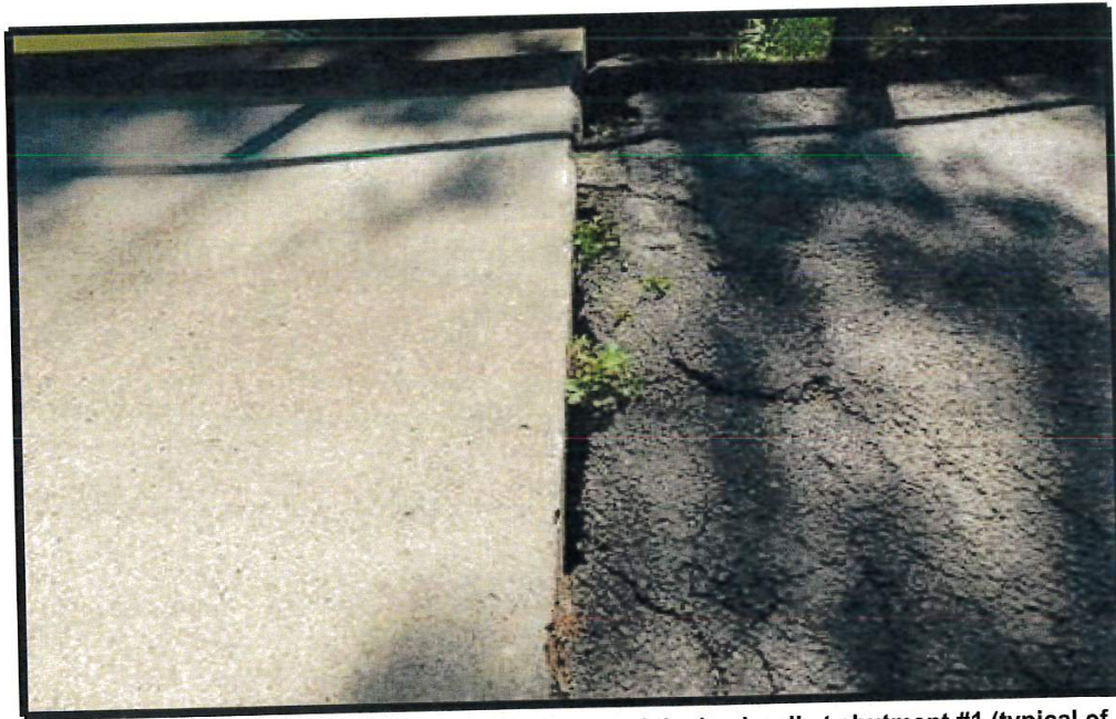
A minor void in the approach between the deck and the backwall at abutment #1 (typical of abutment #2).
