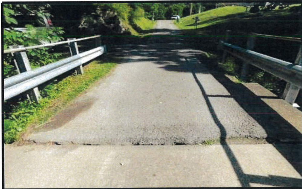
Condition of the approach at abutment #2, with moderate cracking and light spalling.
