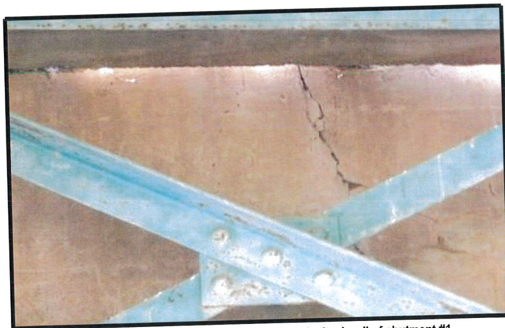
An 1/8" vertical crack, with light spalling, in the backwall of abutment #1.
