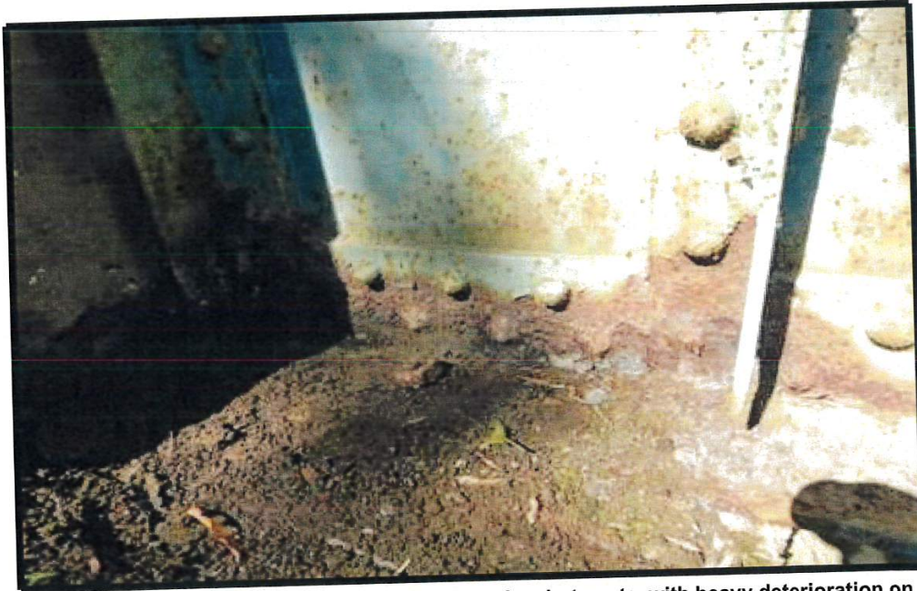
Moderate to heavy rust on the steel elements at the abutments, with heavy deterioration on the bearing bolts (downstream girder at abutment #1 shown).
