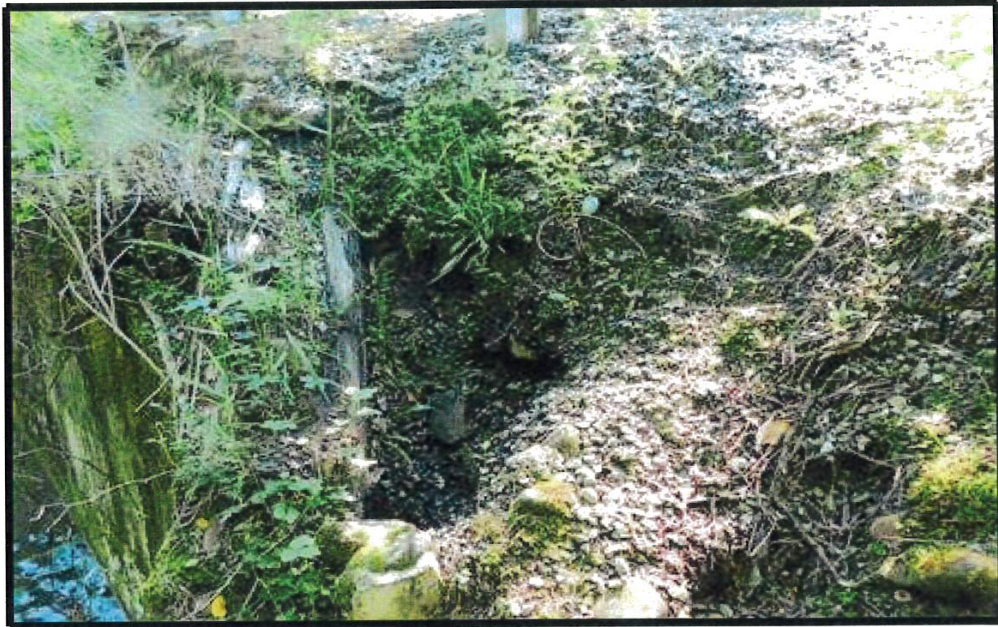
Moderate shoulder erosion behind the upstream wingwall of abutment #1.
