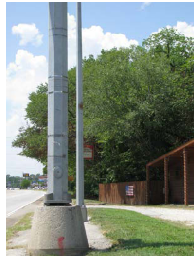
Image 7. Traffic signal obstructing the pedestrian zone on Highway 50 at Oak Street.
