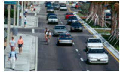
Image 24. Example of a wide outside lane that provides adequate space for cyclists and motor vehicle users to operate side-by-side. (Source: bicyclinginfo.org )
