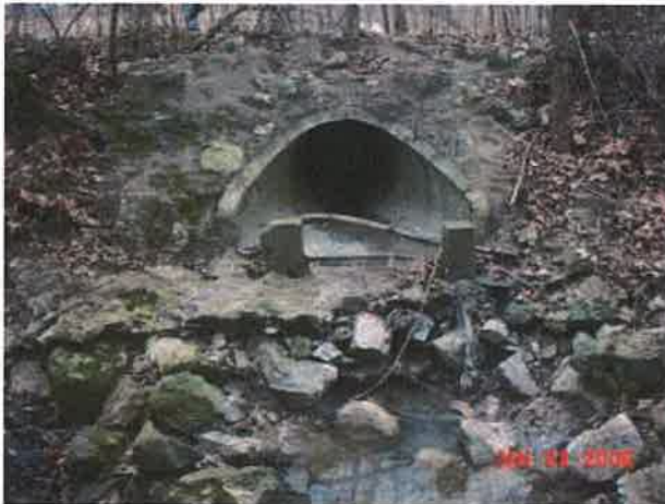
Figure 3: Storm sewer outfall
