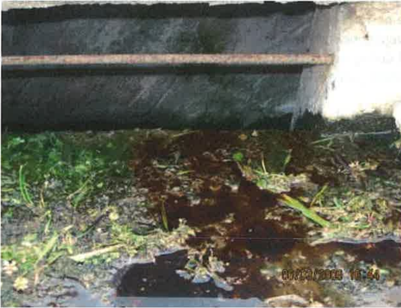
Figure 6: Presence of Commercial Illicit Discharge-grease from restaurant
