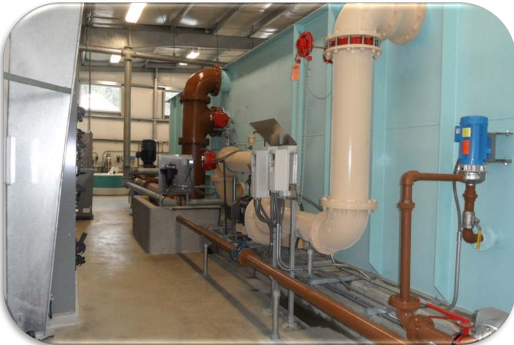
FIGURE 5.3.8 COOPER CREEK WTP FILTER UNIT AND PIPING
