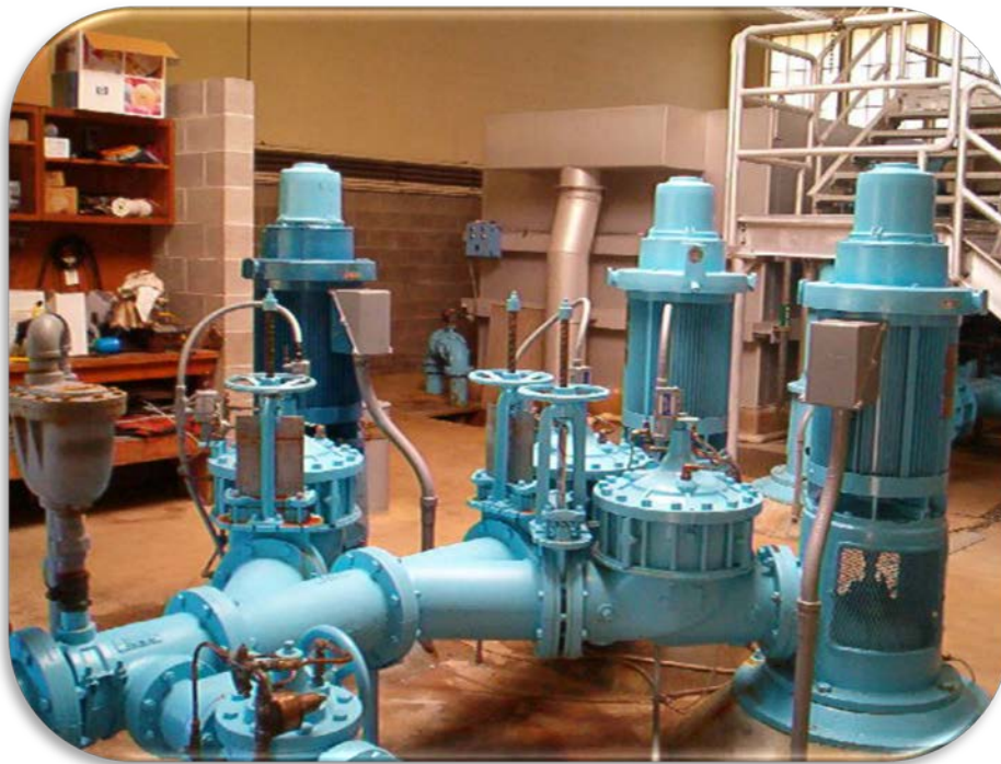
FIGURE 5.3.4 NONPAREIL WTP TREATED WATER PUMPS
