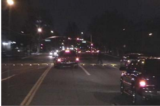
Figure 10-2. In-Pavement Lights
