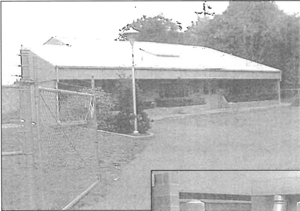
Nonpareil Water Plant
