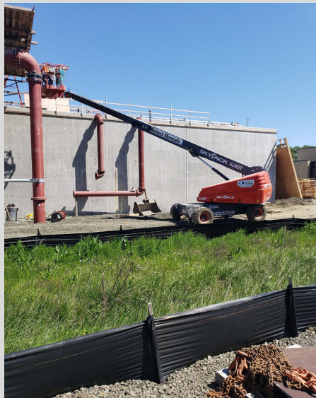
Installation of mechanical piping at the influent end of the SBR and Headworks.
