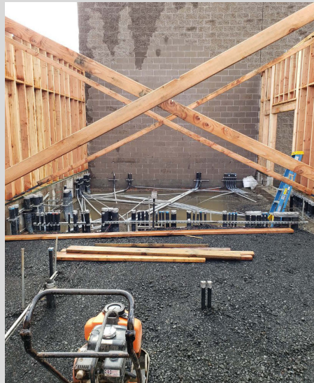
Completed installation of electrical conduits within the electrical room of the new Control Building.
