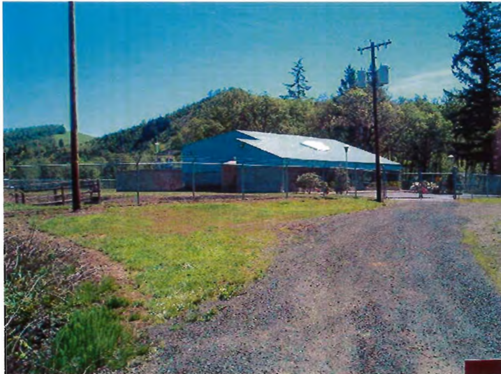
FIGURE 5.3.2 NONPAREIL WTP BUILDING
