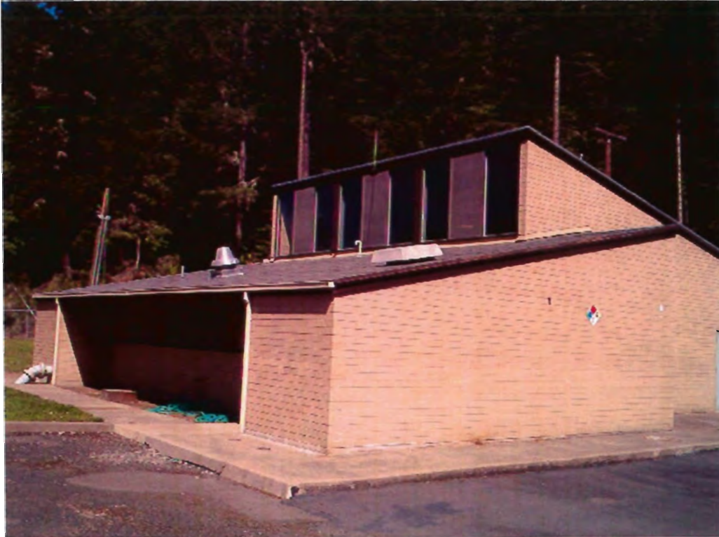
FIGURE 5.3.6 COOPER CREEK WTP BUILDING
