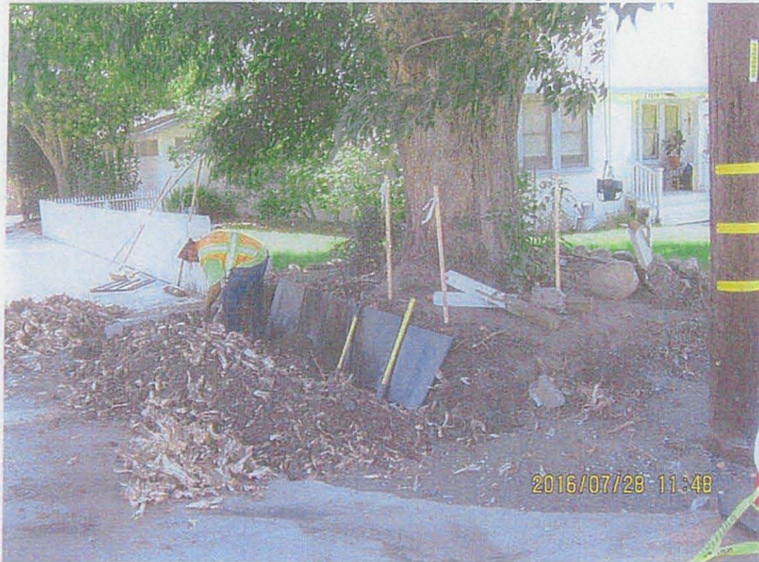
Below Shamel ash installing root barriers after root pruning
