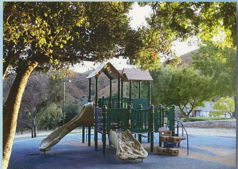
Eagle View Park Playground Reconstruction
