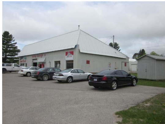
LeRoy Garage, LeRoy, Michigan
