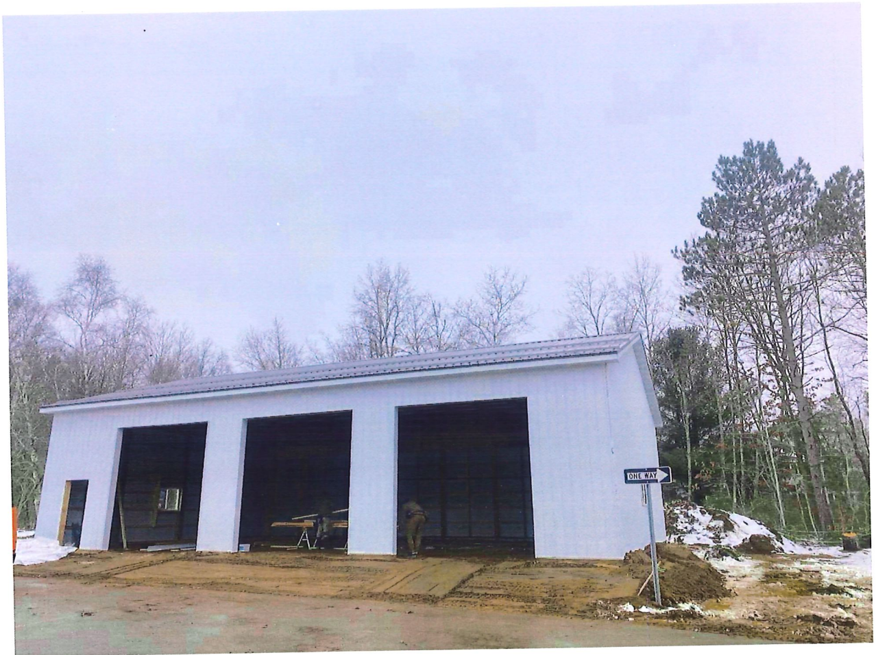
Cherry Grove Fire Department Barn (Progress Photo)
