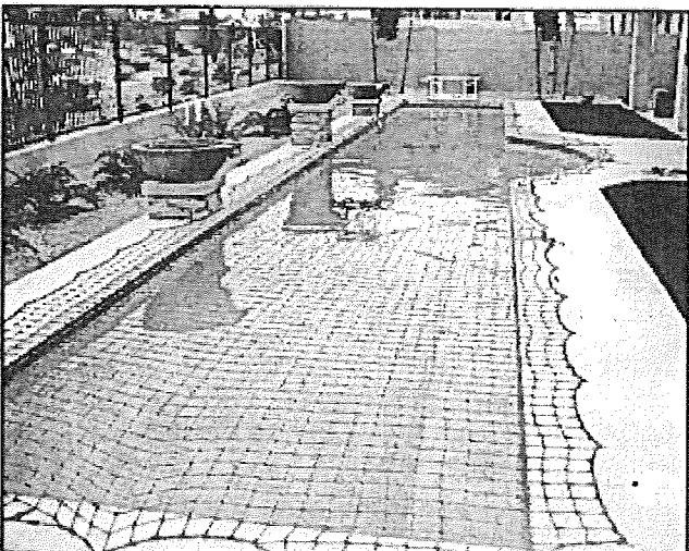
FIGURE 305.1(4) NONPOWERED MESH COVER DOES NOT ALLOW FOR ABSENCE OF BARRIER AROUND POOL
