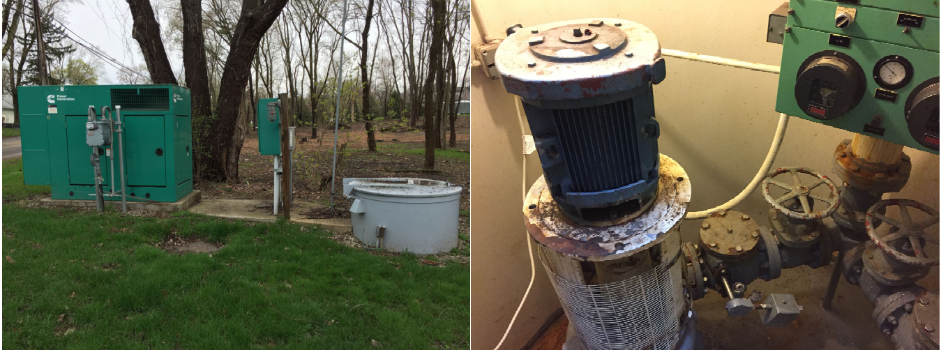
Figure 8-12. East Shore 2 Pump Station Site View and Corrosion in Dry Pit
