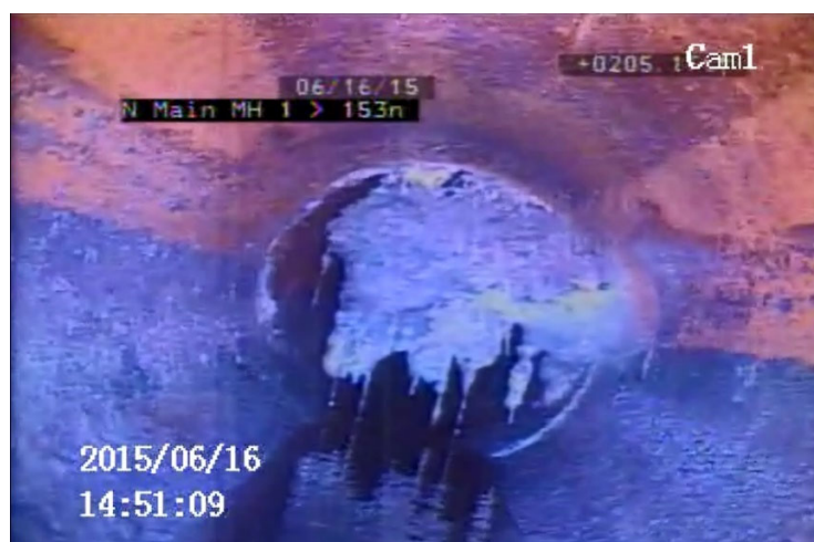
Figure 8-9. Root Intrusion under North Main Street
