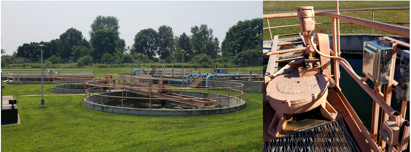
Figure 8-19. Final Settling Tanks
