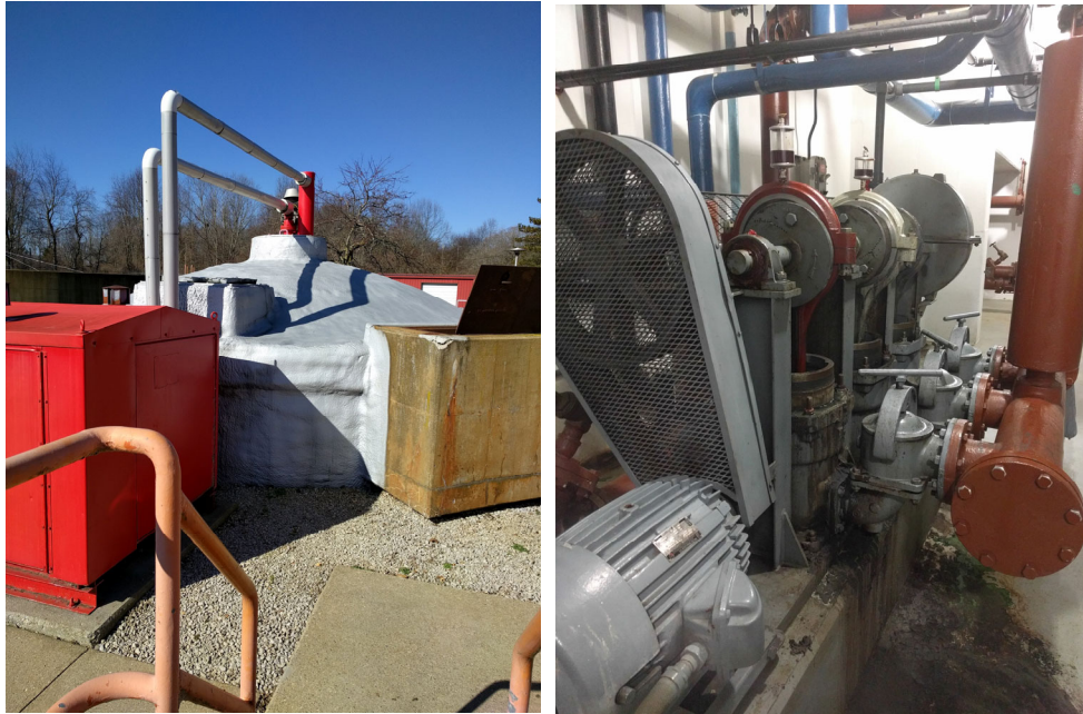
Figure 8-23. Anaerobic Digester and Triplex Sludge Pump
