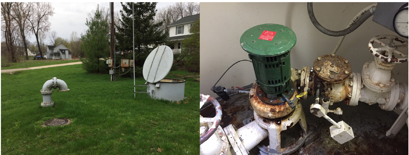
Figure 8-7. Main Street Pump Station Site View and Pump, Discharge Piping and Valve Corrosion
