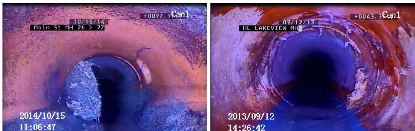
Figure 3-1. Grade 3 Defect vs. Grade 4 Structural Defect
