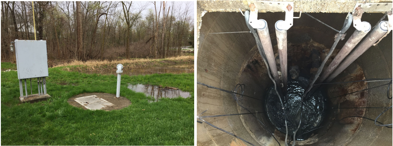
Figure 8-16. North Shore 2 Pump Station Site View and Corrosion/Infiltration in Wet Well
