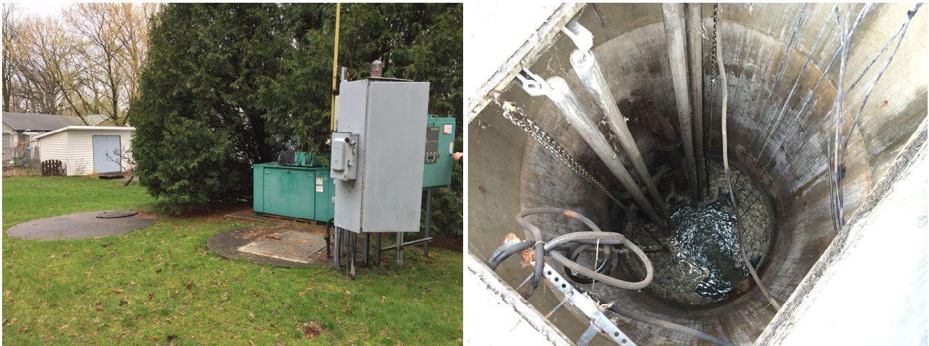
Figure 8-17. Horseshoe Lake 2 Site View and Wet Well Infiltration and Discharge Piping Corrosion
