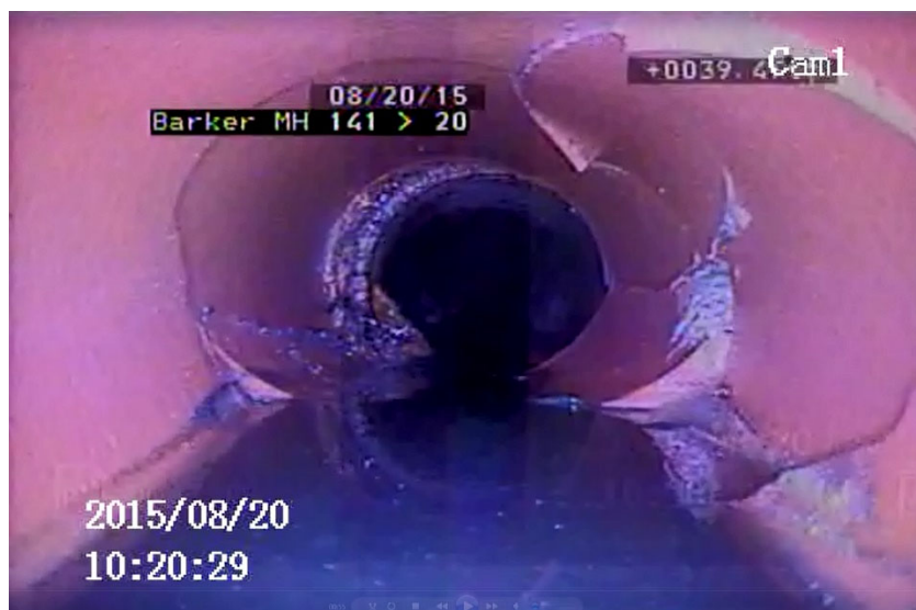
Figure 8-6. Broken Sewer under Barker Road
