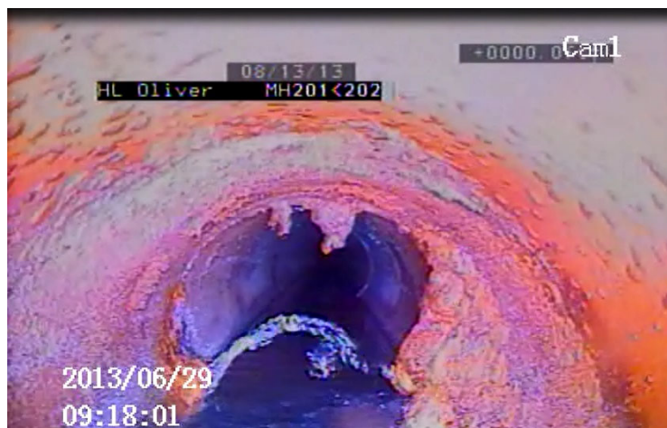
Figure 8-8. Gushing Infiltration and Encrustation Under Oliver Boulevard
