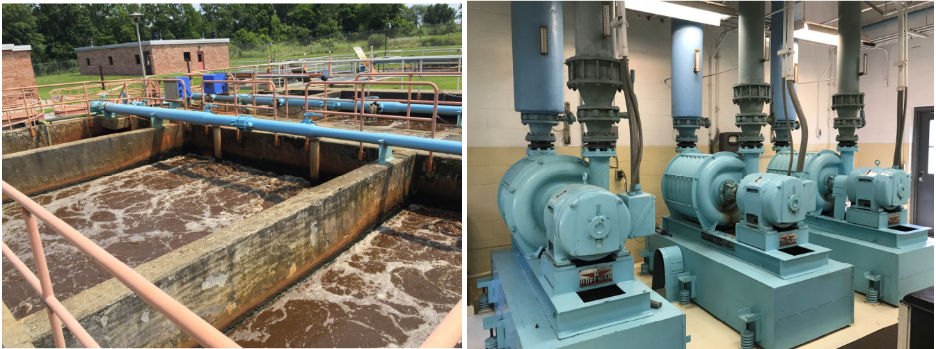
Figure 8-18. Aeration Tanks and Blowers
