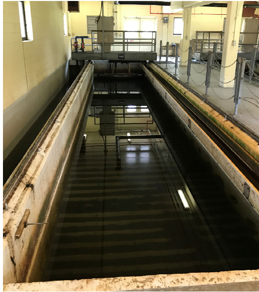
Figure 8-25. Existing Traveling Bridge Filter
