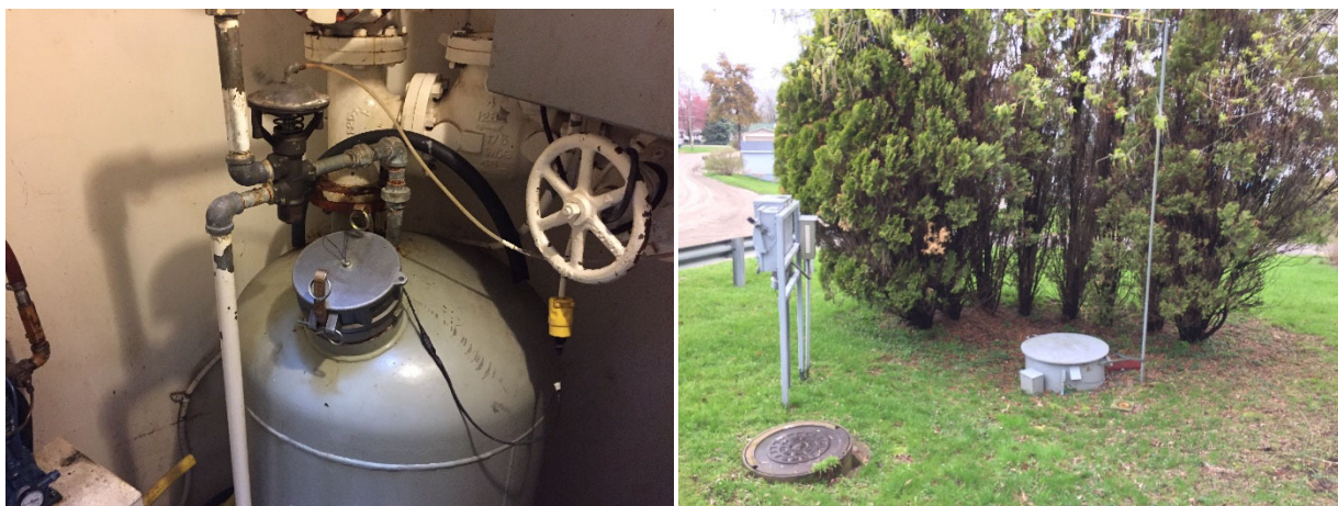
Figure 8-13. North Shore 1 Pump Station Site View and Ejector Pumps
