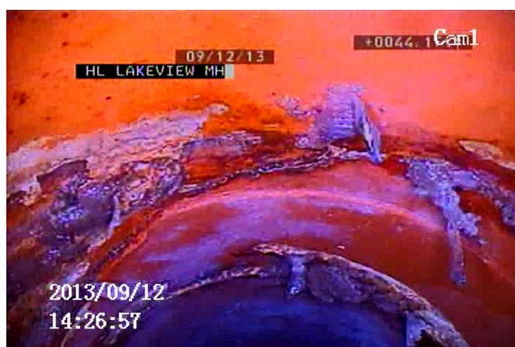
Figure 8-10. Multiple Fractures under Lakeview Drive
