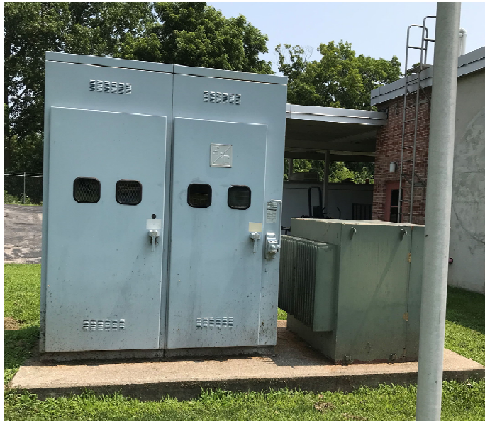
Figure 8-21. Primary Switchgear
