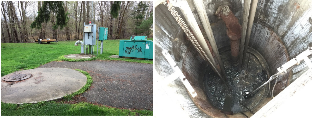
Figure 8-14. Horseshoe Lake 1 Pump Station Site View and Corrosion/Infiltration in Wet Well
