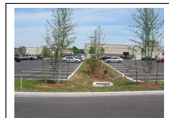
Landscaped parking lot islands can also serve as vegetated swales for storm water drainage.
