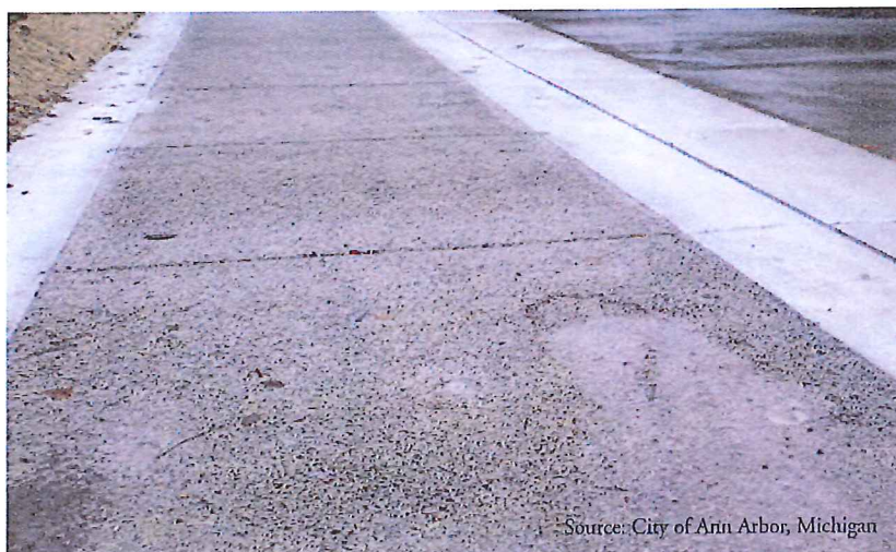
Completed permeable concrete alley.
