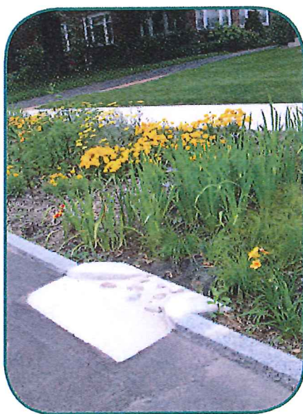
Energy dissipater between road and bioretention.
