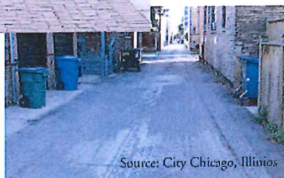
(Above) Permeable block alley after reconstruction and (right) before reconstruction.
