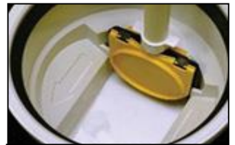
Installing a backwater valve prevents sanitary backups during heavy rain events.
