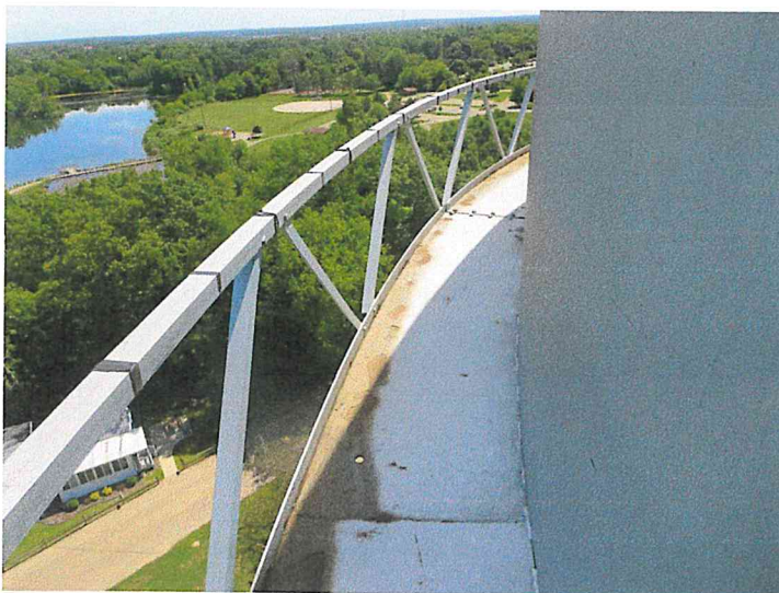
15) The balcony and handrail are in good condition overall.
