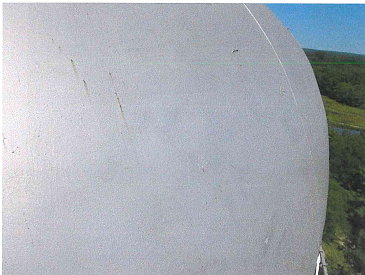
18) The roof knuckle is in good condition.
