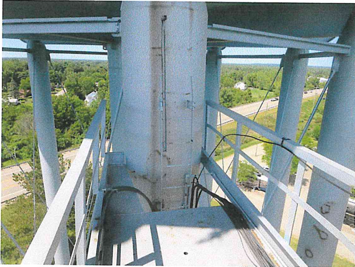
13) The platform at the top of the leg is in good condition.
