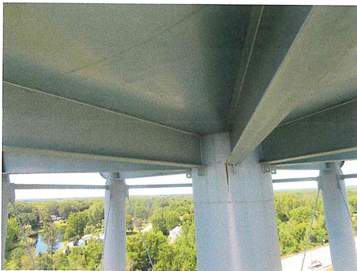
12) The radial arm beams are in good condition.
