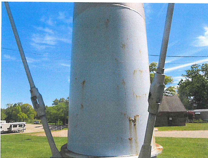
9) The sway rods and turnbuckles are in good condition.
