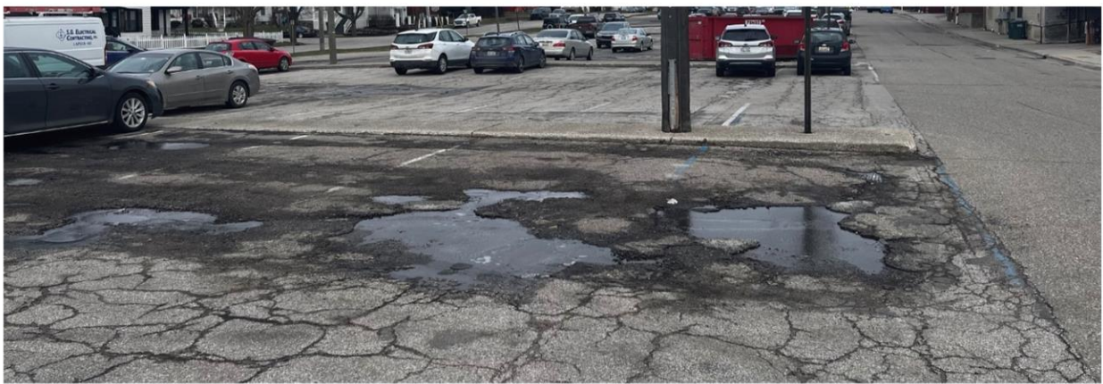
Parking Lot 9 Pavement Deterioration
