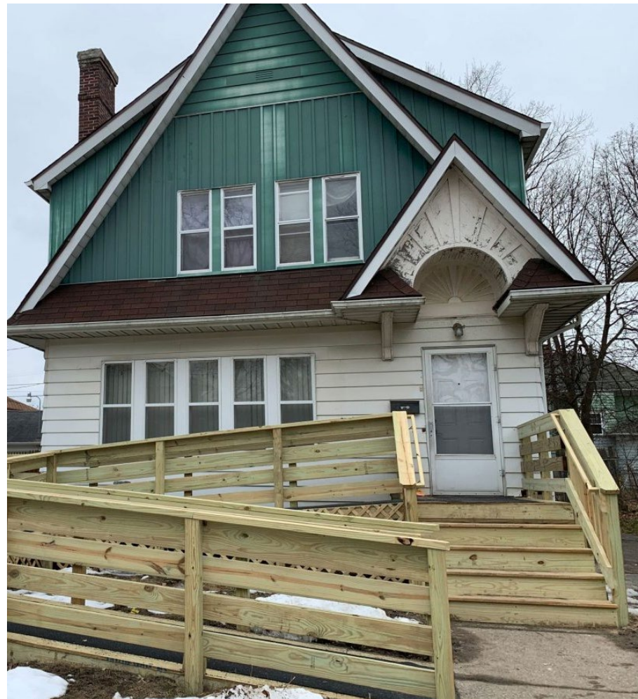
Source: Habitat for Humanity
