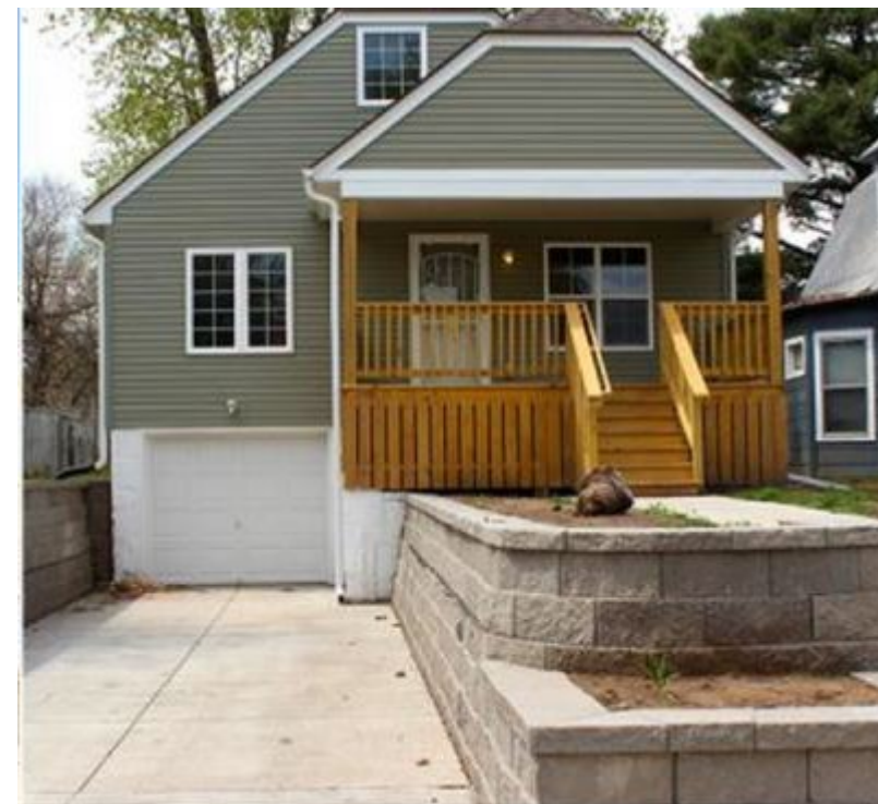
Source: Habitat for Humanity
