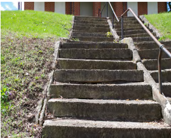
Left: The steps leading to 410 E. Capitol Avenue are sagging, uneven, and deteriorated.
