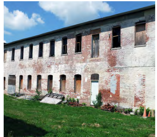
Right: 100 Lafayette is missing the rear windows allowing the weather to penetrate into the structure.
