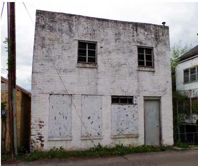
Above: 504 E. Capitol has boarded up/deteriorated windows and severe step cracking.
