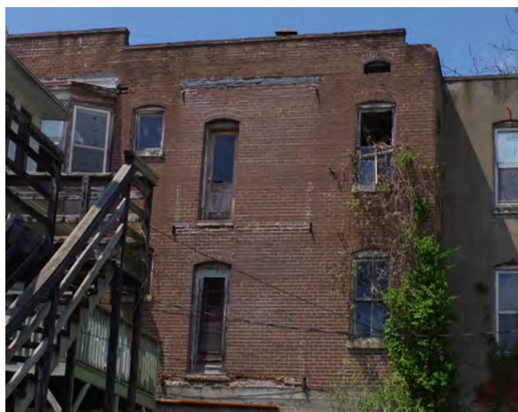
Left: 519 E. Capitol is boarded-up and vacant. The windows, doors, exterior walls, and roof are all severely deteriorated.
