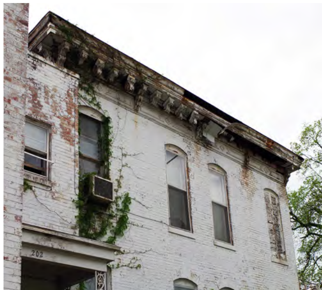
Above: 528 E. Capitol is a former single-family home that has been converted into a multi-family. The soffit, fascia, gutters, windows, and bricks on this building are deteriorated.
