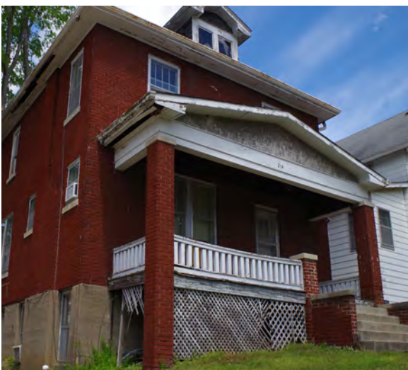
Left: The soffits, fascia, porch, and gutters on 214 Jackson are deteriorated. Downspout is missing.
