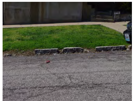
Right: A deteriorated curb and gutter along Marshall.
