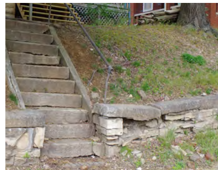
Below: The steps and retaining wall at 617 E. High are deteriorated and the retaining wall is failing.
