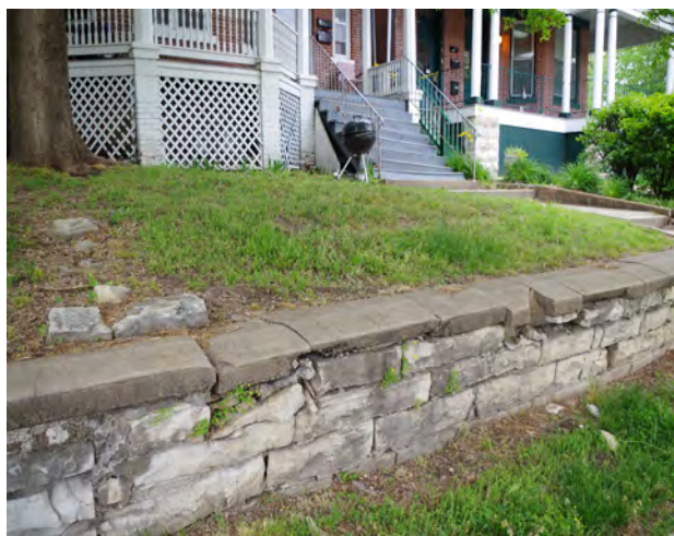
Above: The retaining wall in front of 527 E High is deteriorated.
