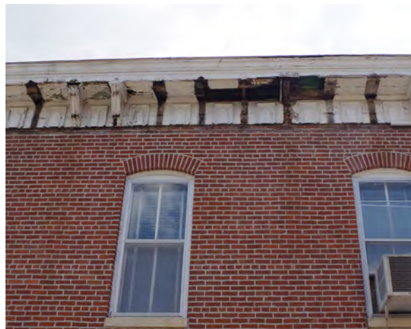
Left & Right: The gutters, downspouts, soffit, and fascia are deteriorated on 507 E. Capitol.
