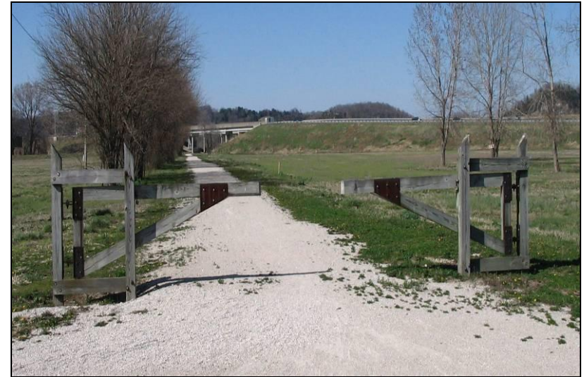
Typical stone dust trail construction at the Katy Trail
