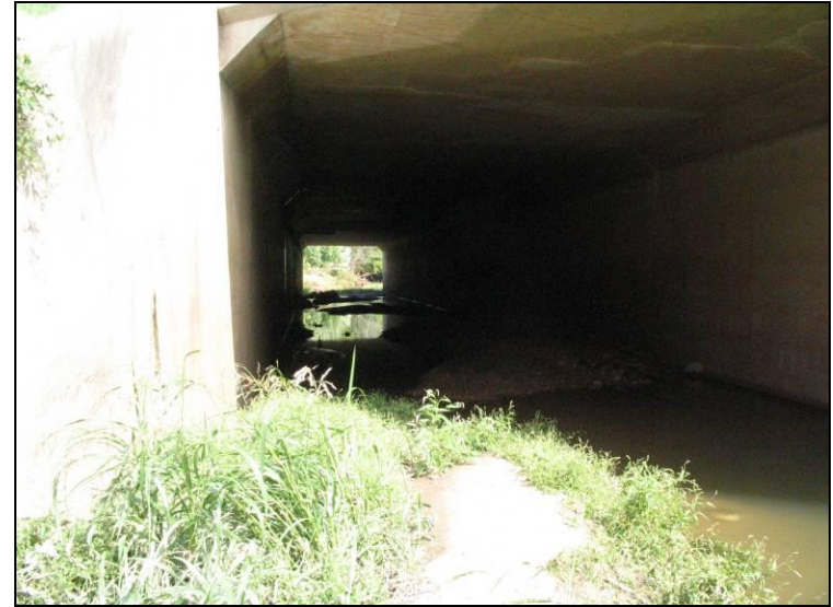
The box culvert under Highway 50 and Missouri Boulevard
