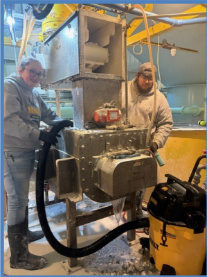
Left: Brooke and Alex clean out the slaker. The slaker combines lime and water and is the first step in the water softening process.
