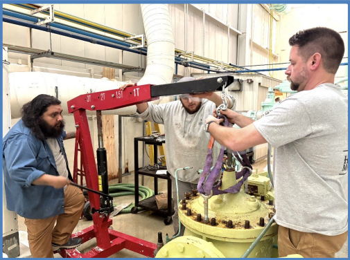
Below: Stevie (left), Alex (center), and Daniel disassemble the pressure reducing valve for cleaning.
