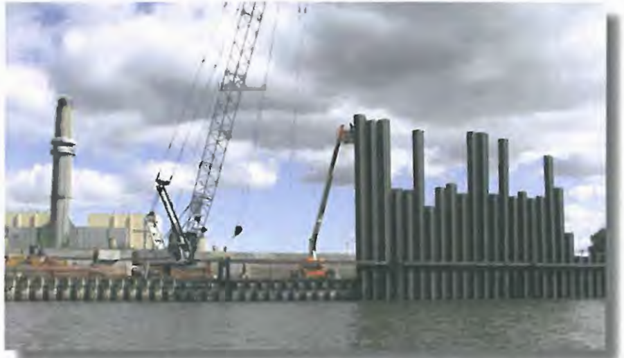
$21-million seawall reconstruction along the Saginaw River in Bay City.
