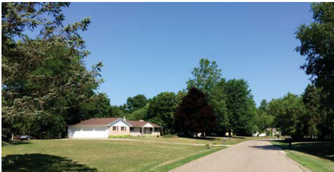
Single Family Suburban Residential Neighborhood
