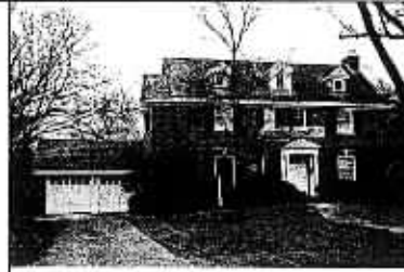
835 S. WASHINGTON STREET Giles House Colonial Revival 1933 Oliver, Ralph
