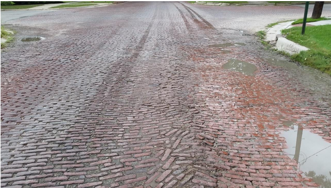
04. Looking at broken bricks and ponding water.
