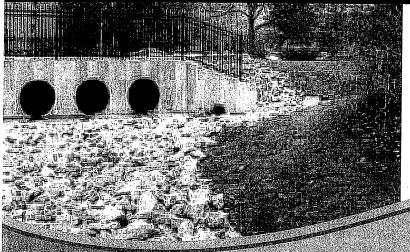
This project included design and re-construction of the Sawmill Creek culvert crossing and concrete spillway at Walnut Drive that failed in severe storm events in 2008 - 2009 and resulted in the collapse of the roadway.
