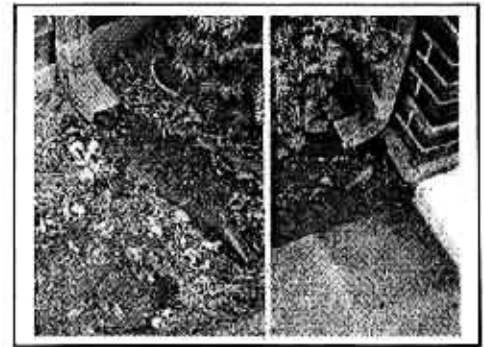
Image 23a & b: Existing and missing splashblocks
