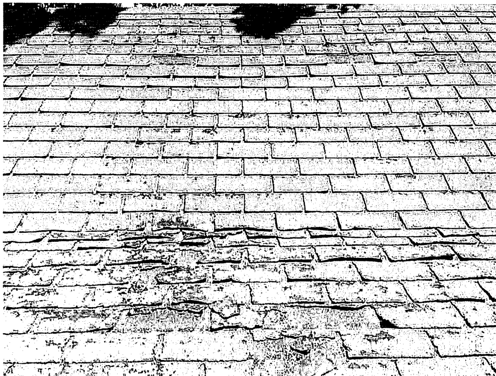
#14 -- Section A: Overview showing deteriorated and missing shingles. [1603806R0014.jpg]
