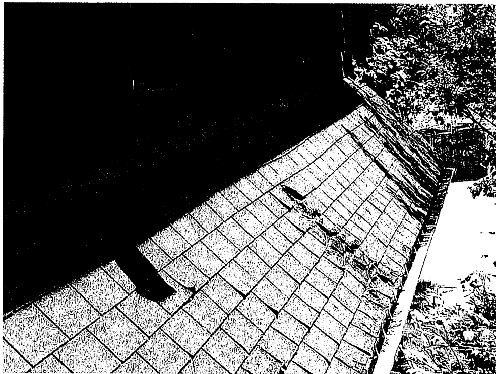
#7 -- Section A: Overview facing south showing deteriorated shingles. [1603806R0007.jpg]
