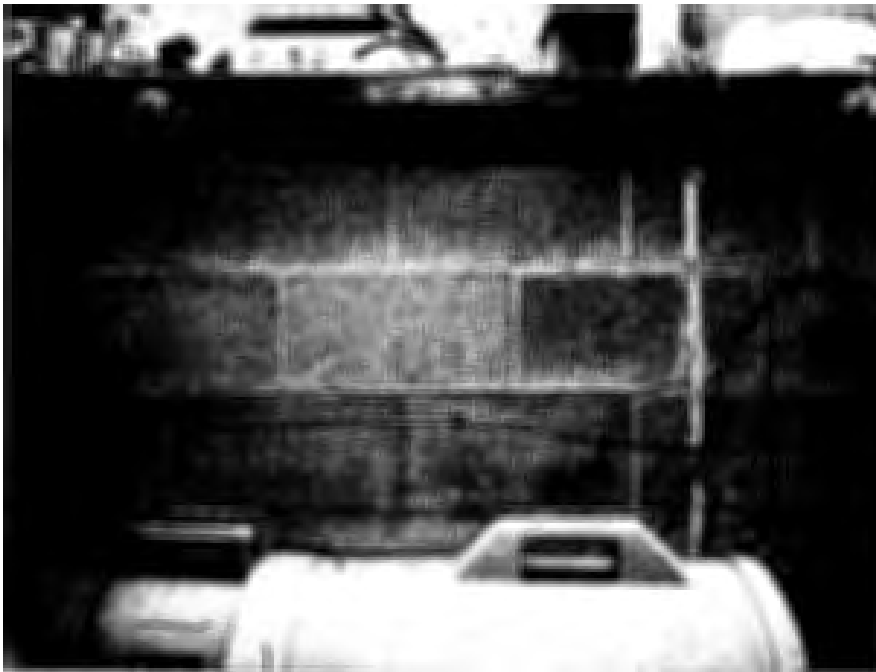
5. West Wall Horizontal Crack in CMU
