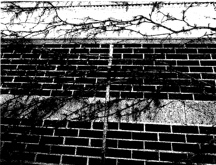
3. North Wall Control Joint (Exterior view)
