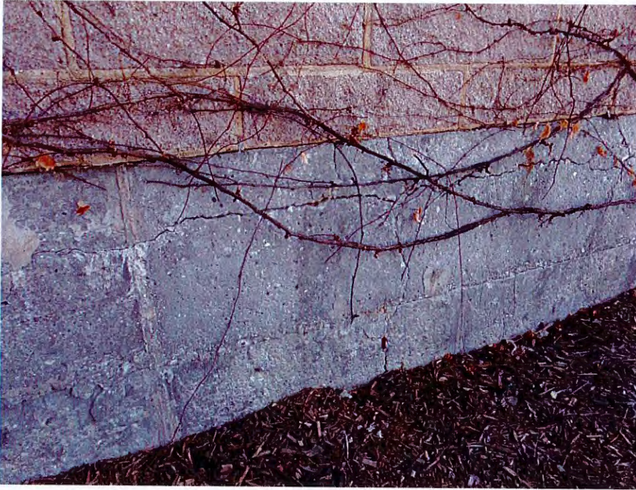
12. Horizontal crack top of tank wall West Exterior Elevation
