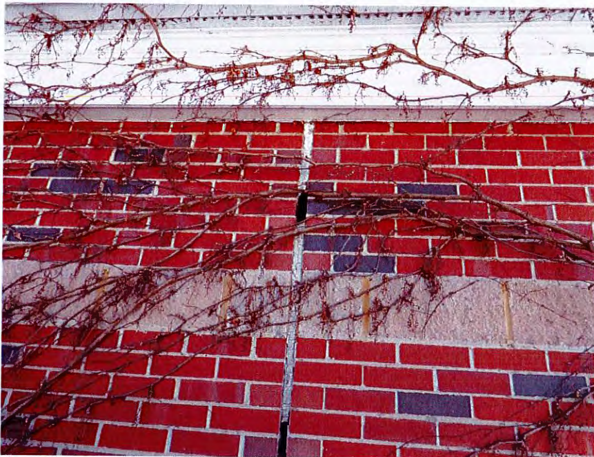
3. North Wall Control Joint (Exterior view)
