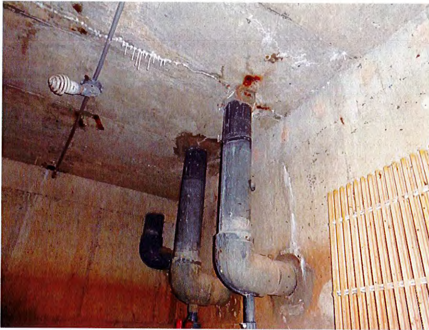
10. Rigid Pipe Connection through west wall
