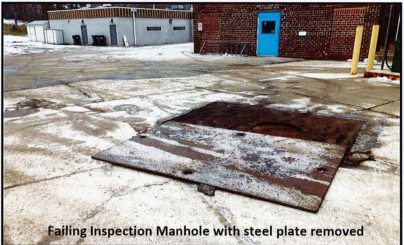
Steel Plate covering Failing Inspection Manhole
