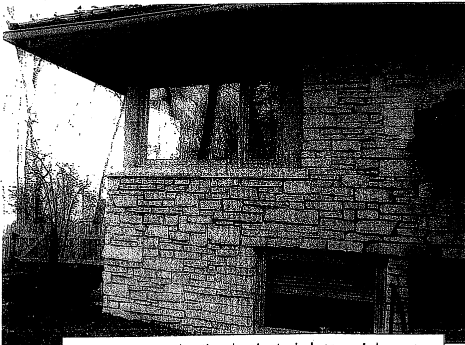
Northeast corner elevation showing typical corner window, basement windows, stone work and deep eaves with tongue and groove cladding on the eaves.
