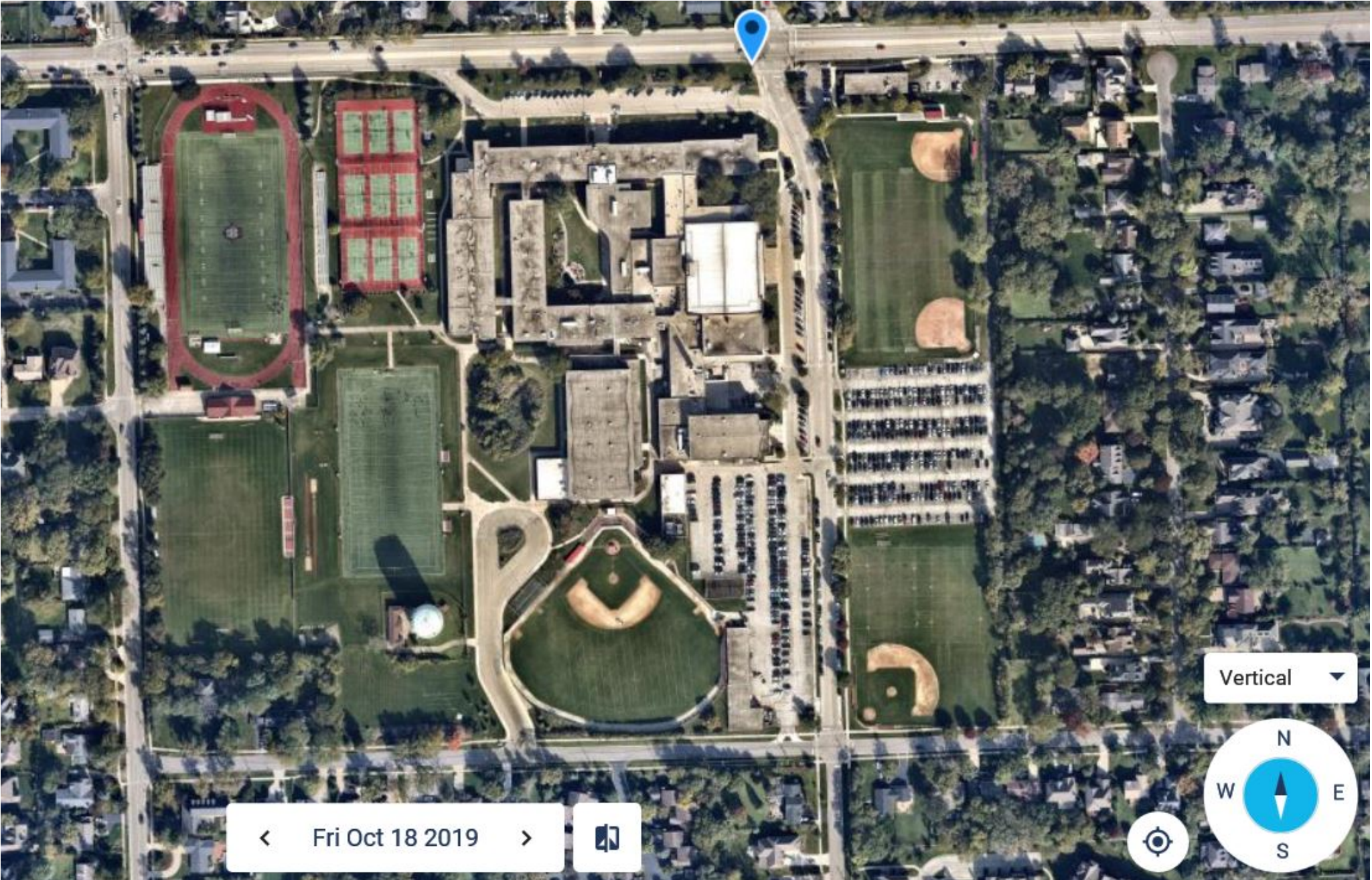
Attachment 4: Aerial View of Hinsdale Central High School Campus, 5500 S. Grant St.
