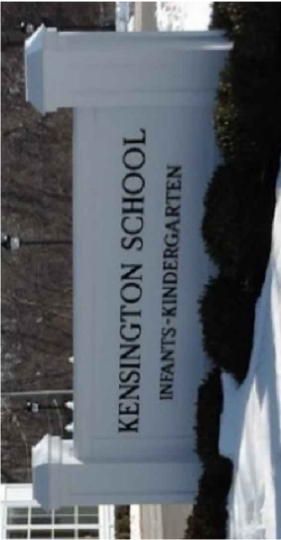
GROUND SIGN: 8" x 6" SURFACE MOUNTED BLACK LETTERS NON ILLUMINATED
