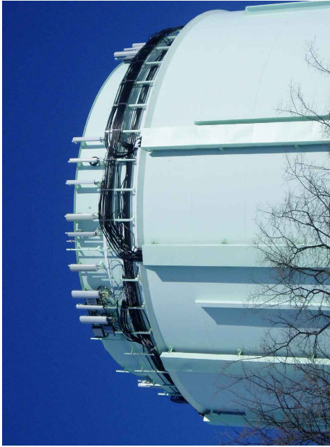
11 COAX ROUTING &amp; ANTENNA SECTOR
