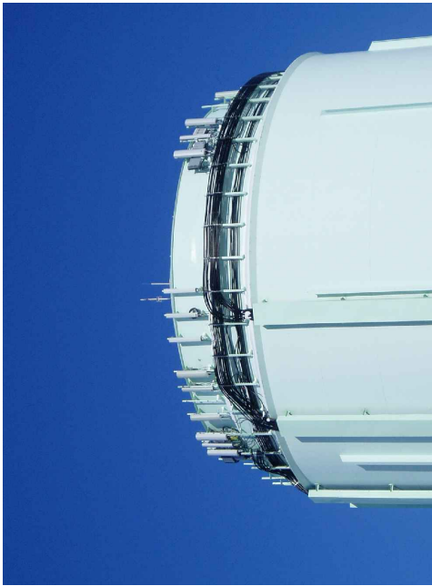
COAX ROUTING & ANTENNA SECTOR
