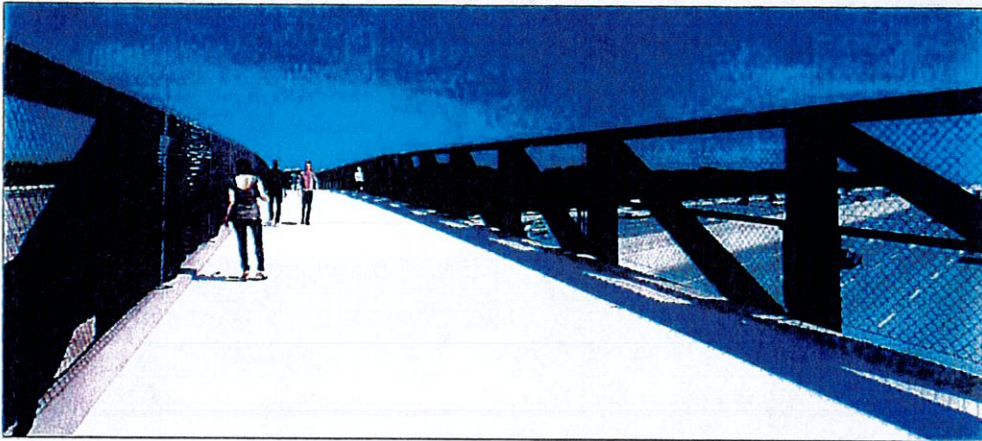
Handrail, safety rail and galvanized chain link
