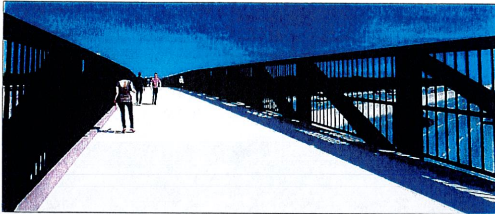
Handrail, safety rail and vertical pickets
