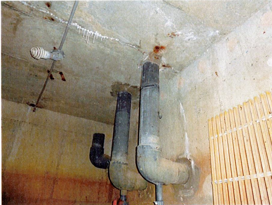
10. Rigid Pipe Connection through west wall
