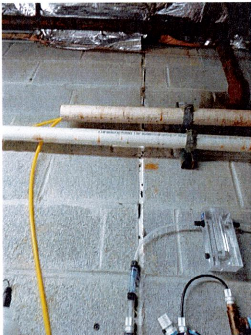
6. West Wall Control Joint
