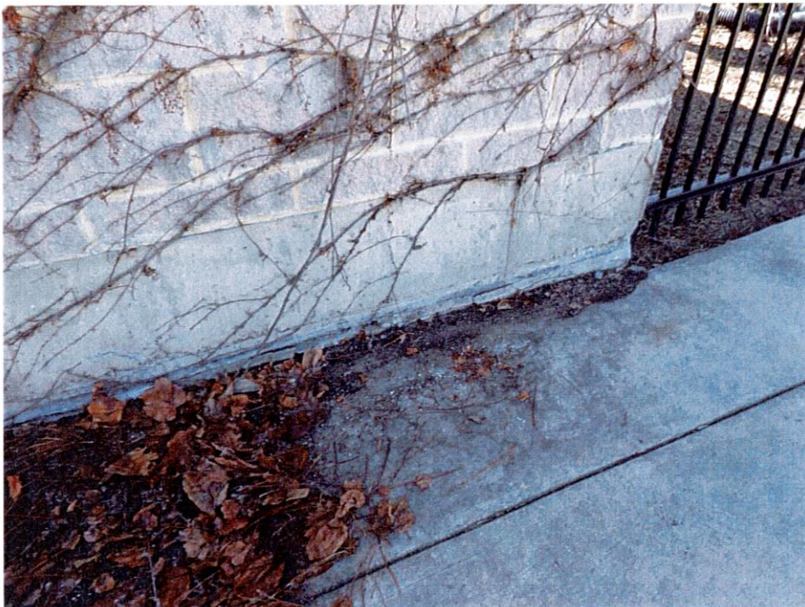
11. Pool slab depressed north west corner of building
