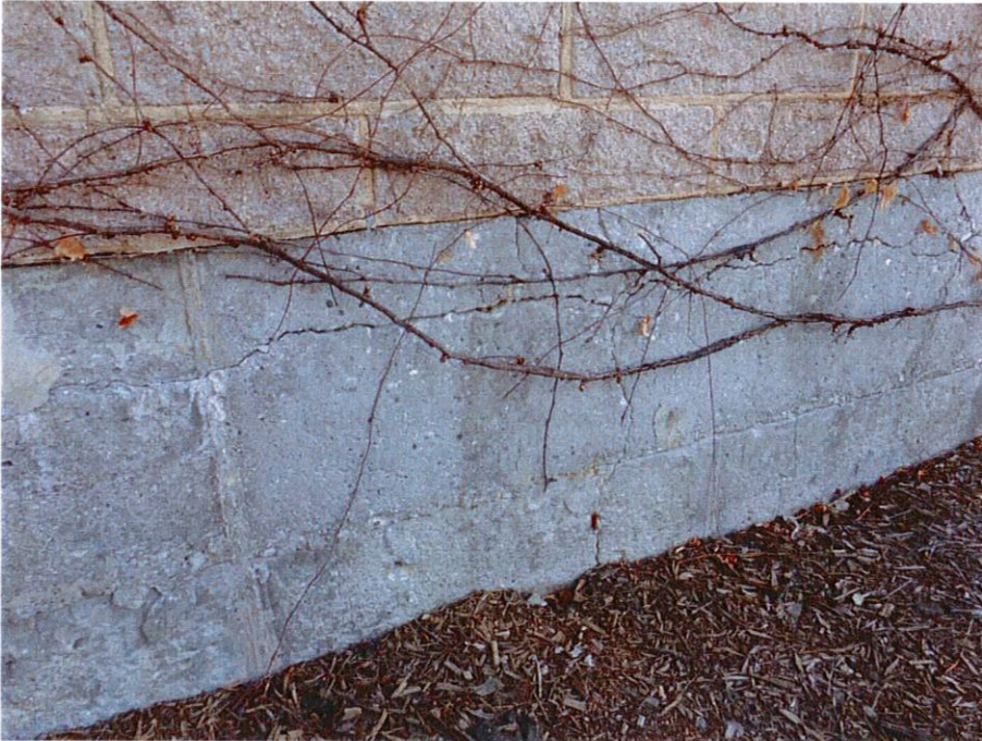
12. Horizontal crack top of tank wall West Exterior Elevation
