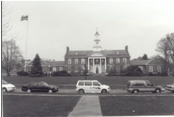
Figure 1: Hinsdale Memorial Building
