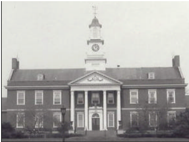
Hinsdale Memorial Building
