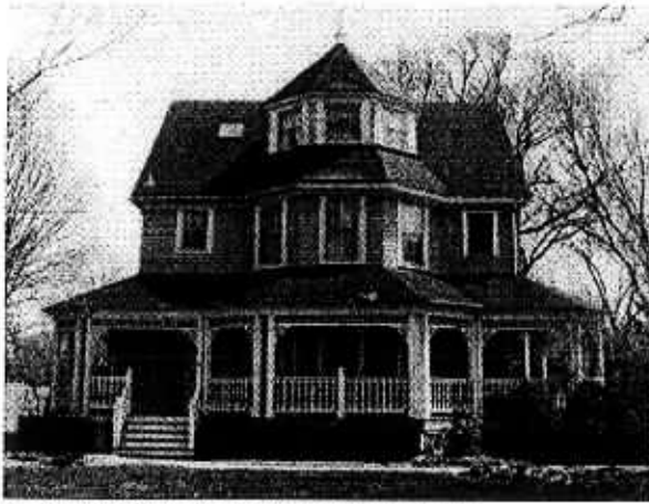
W. H. Edwards House, 315 S. Washington Street
