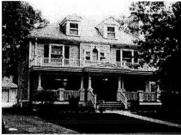
Garry W. Munson House, 515 S. Lincoln Street
