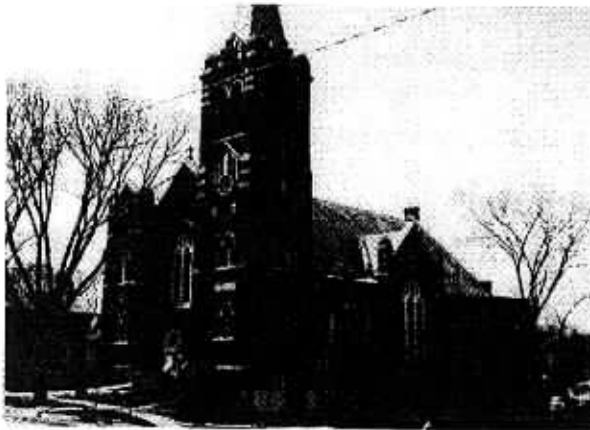
Zion Lutheran Church, 204 S. Grant Street
