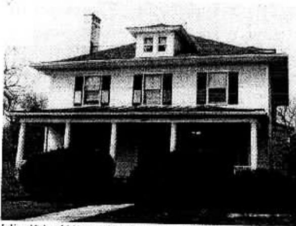
Julian Hulanski House, 304 S. Washington Street
