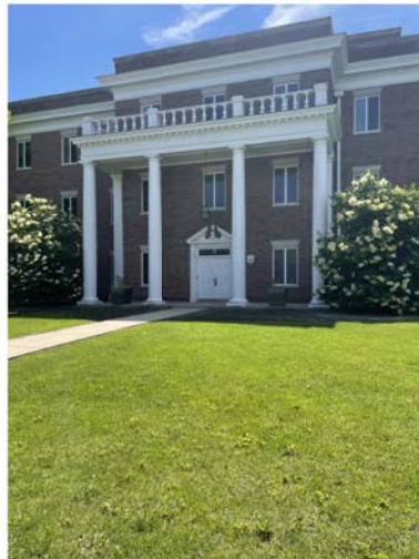
PORTICO TO BE REMOVED DUE TO WOOD DETERIORATION. EXISTING DOOR TO BE REPLACED WITH NEW THERMALLY BROKEN ALUMINUM DOOR. SEE ARCHITECTURAL PLANS AND ELEVATIONS.
