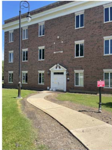
TYPICAL FOR NORTH AND SOUTH ELEVATIONS. EXISTING DOOR TRIM TO BE REPLACED WITH NEW CANOPY. SEE ELEVATIONS FOR NEW SCOPE OF WORK. EXISTING DOOR TO BE REPLACED WITH NEW INSULATED METAL DOOR.
