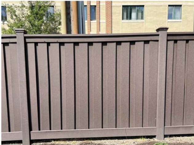
PRIVACY FENCE SHALL SCREEN TRANSFORMER LOCATED NORTH OF EAST BUILDING ENTRANCE. THE FENCE IS BEING PROPOSED DUE TO LIMITED SPACE THAT WILL NOT ACCOMMODATE A VERTICAL EVERGREEN HEDGE. FENCE SHOWN IS MANUFACTURED BY TREX- STYLE - SECLUSIONS AT 8' HEIGHT. MATERIAL - COMPOSITE. COLOR - WOODLAND BROWN.
