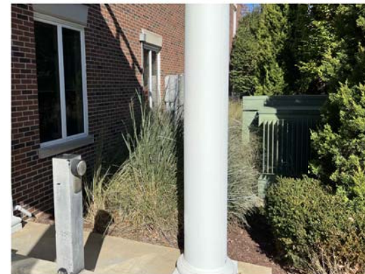
SPACE BETWEEN PORTICO AND TRANSFORMER IS LIMITED WITH ~4' NARROW GREEN SPACE, OF WHICH 3' IS REQUIRED FOR PERIMETER CLEARANCE, LEAVING INSUFFICIENT ROOM FOR A VERTICAL EVERGREEN HEDGE. LANDSCAPE TO BE REPLACED WITH SOLID PRIVACY FENCE, CLIMBING VINES, AND APPROPRIATELY SIZED PLANTINGS. SEE LANDSCAPE PLAN AND NEW TRANSFORMER SCREEN.
