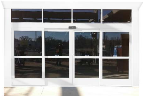
EAST DOOR SHALL BE REPLACED BY NEW ALUMINUM AND GLASS SLIDING DOORS, TRANSLUCENT TRANSOM GLASS AND FRAME, SIMILAR TO ABOVE IMAGE. PROVIDE WHITE POWDER COAT TO ALUMINUM DOOR AND FRAME. DOOR TRIM WILL BE SIMILAR TO TRIM SHOWN AROUND DOOR IN IMAGE.
