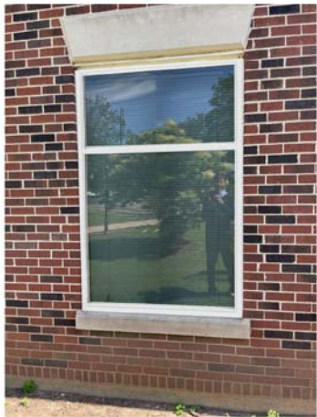
EXISTING WINDOWS SHALL BE REPLACED WITH FIXED THERMALLY EFFICIENT STOREFRONT SYSTEM SIMILAR TO ADJACENT BUILDINGS.
