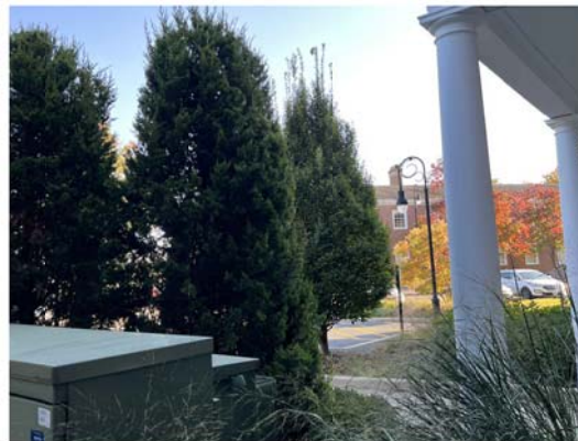
TRANSFORMER IS IN CLOSE PROXIMITY TO MAIN BUILDING ENTRANCE. JUNIPER HEDGE IS OVERGROWN, CREATING NARROW CORRIDOR AT ENTRYWAY AND BLOCKING SECOND FLOOR WINDOWS.
