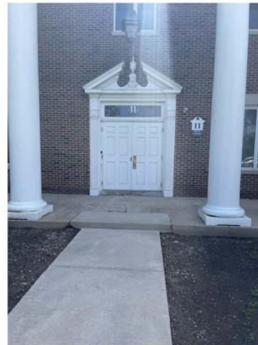
EXISTING DOOR TRIM TO BE REPLACED. SEE ELEVATIONS FOR NEW SCOPE OF WORK. EXISTING DOOR TO BE REPLACED WITH NEW INSULATED METAL DOOR.
