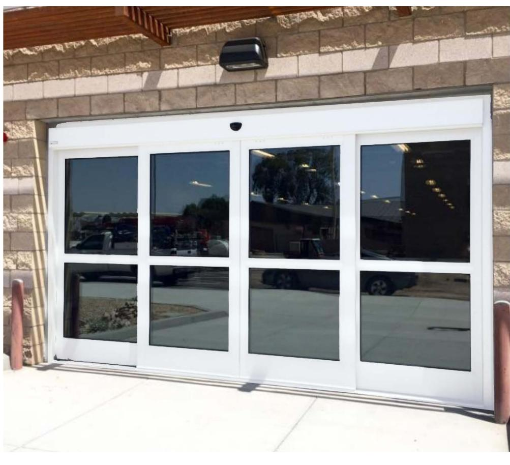
EAST DOOR SHALL BE REPLACED BY NEW ALUMINUM AND GLASS SLIDNG DOORS, TRANSLUCENT TRANSOM GLASS AND FRAME. SIMILAR TO ABOVE IMAGE. PROVIDE WHITE POWDER COAT TO ALUMINUM DOOR AND FRAME.
