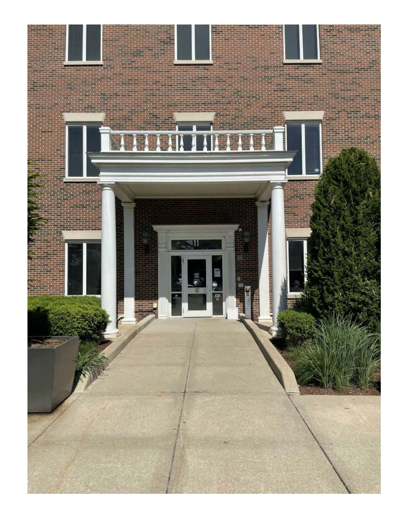
BALUSTRADES TO BE REMOVED DUE TO WOOD DETERIATION. EXISTING DOOR TO BE REPLACED WITH NEW THERMALLY BROKEN ALUMINUM DOOR. SEE ARCHITECTURAL PLANS AND ELEVATIONS.
