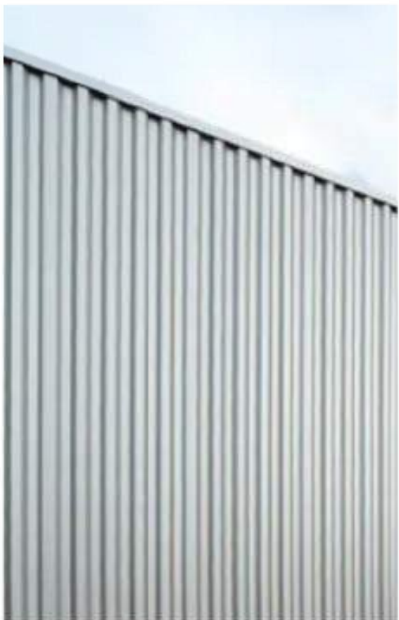
C3 VERTICAL ARCHITECTURAL RIBBED PANEL 1/8" = 1'-0"
