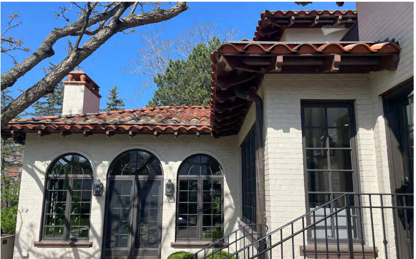
Rear facade - painted brick, window color, clay tile roof, copper downspouts to all match proposed.
