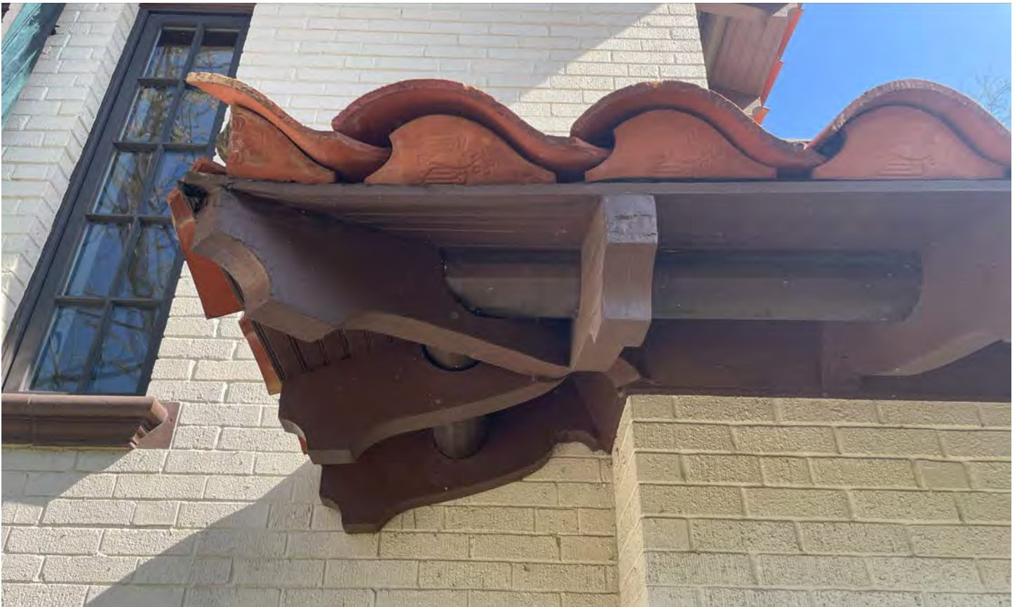
Existing rafter detail to be similar to proposed garage - clay tile roof to match proposed
