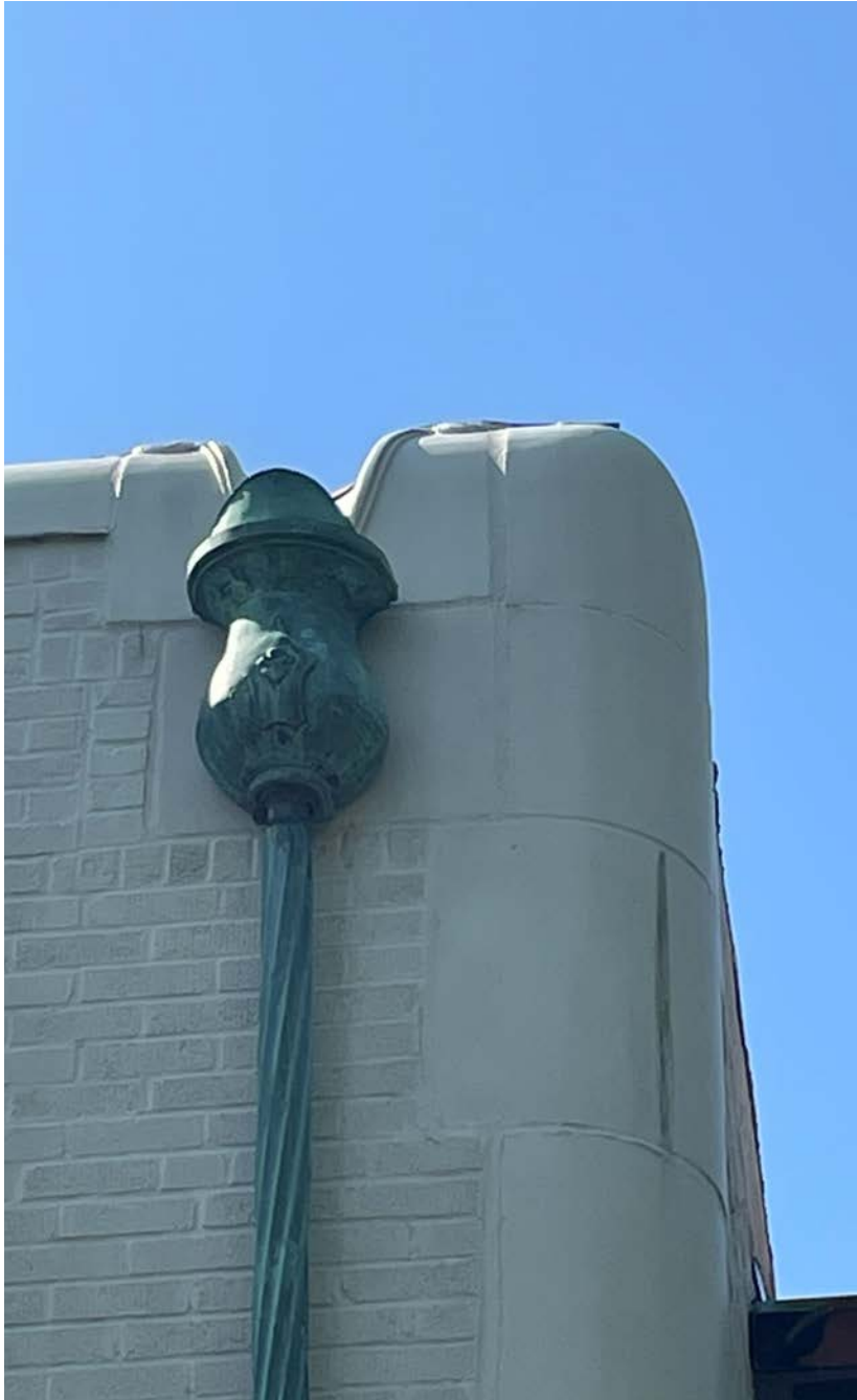
Existing copper collector head to be similar to proposed
