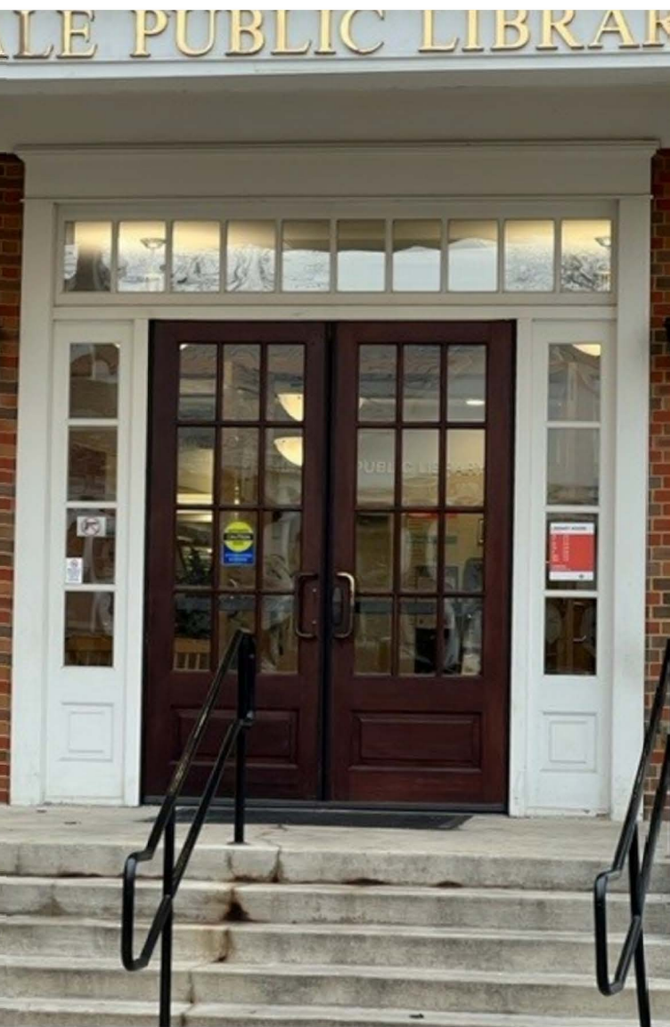
8 existing library door existing photo of library door to be replaced and replicated. Surrounding windows and transom to remain.
