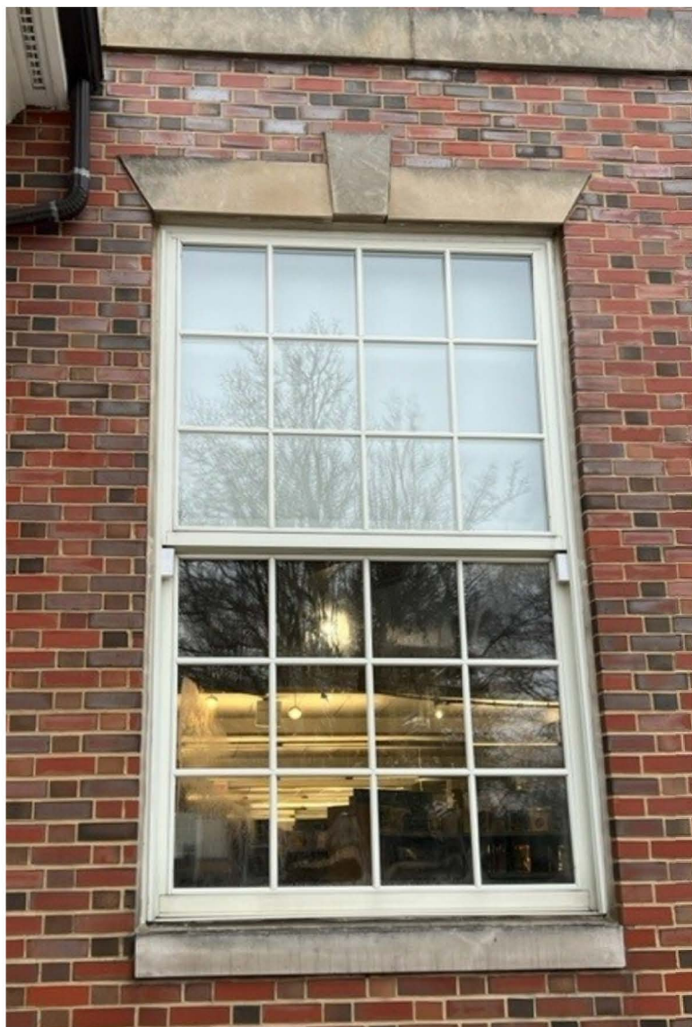
6 existing library window existing double hung aluminum window at library to be replaced
