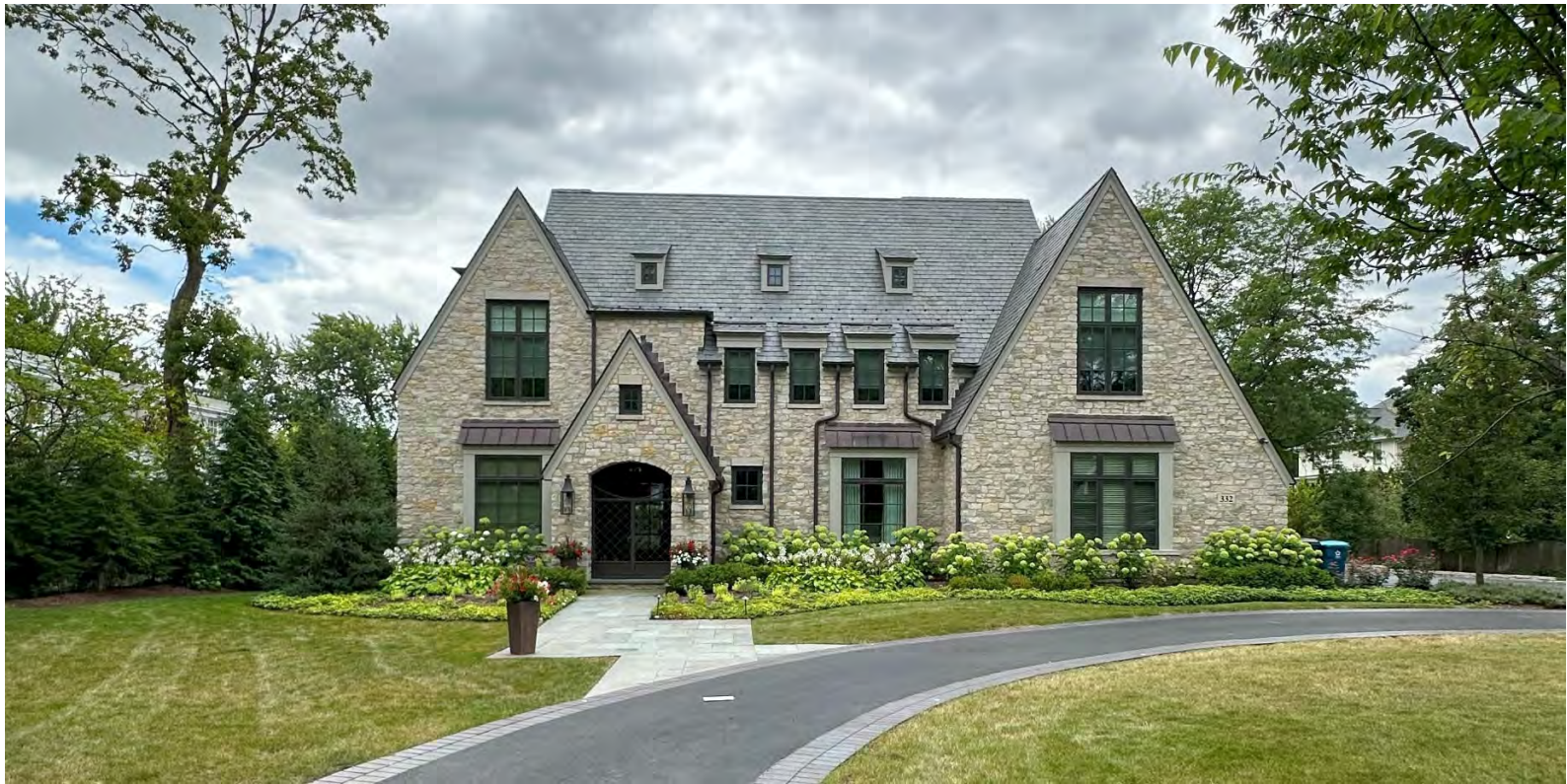
332 E 3rd Street | Home across 3rd street
